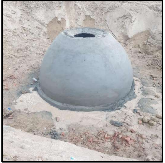
Picture 32: Manhole under Construction
