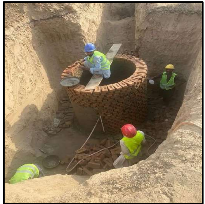
Picture 42: Construction of Manhole is in Progress
