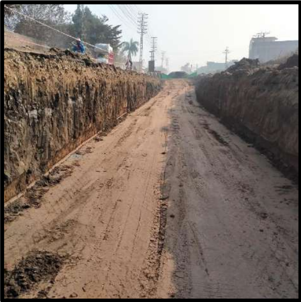
Picture 86: Sewer Bed Preparation
