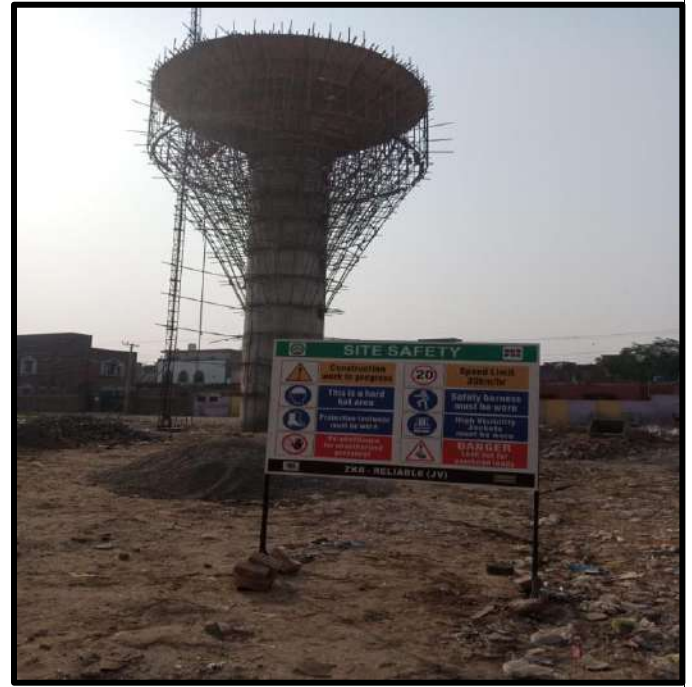
Picture 93: Construction of OHR in Progress
