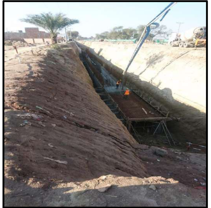
Picture 34: Pouring of Conduit Wall Concrete in Progress
