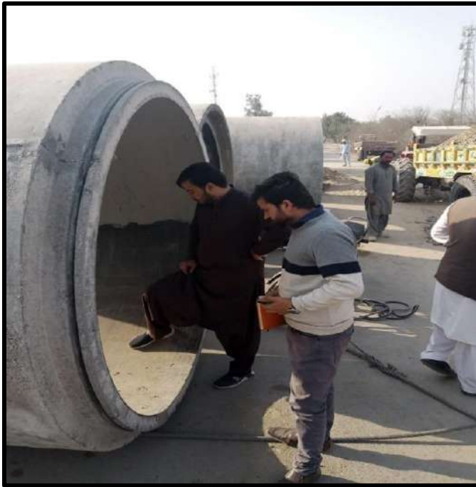
Picture 45: Sewer Checking at Factory
