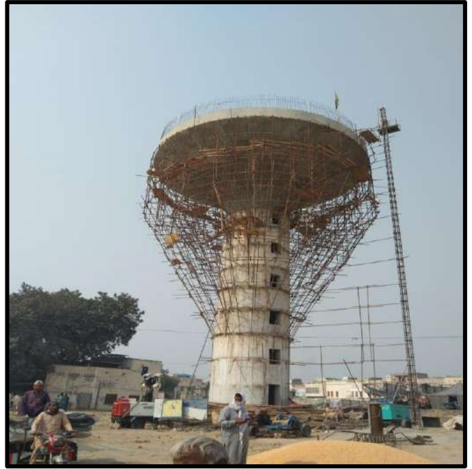
Picture 24: Removing of OHR Shuttering in Progress
