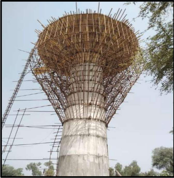
Picture 23: OHR under Construction
