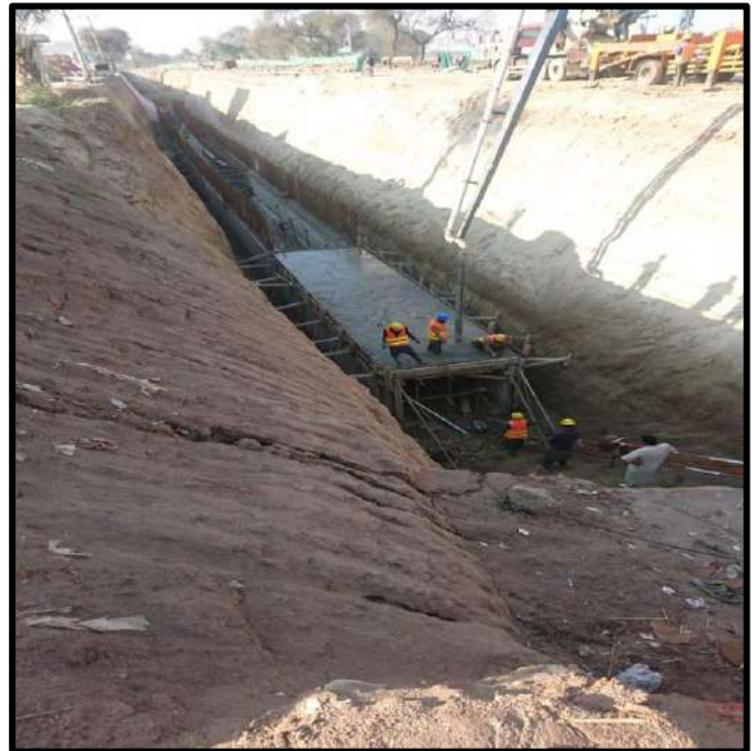
Picture 36: Top Slab Concrete in Progress
