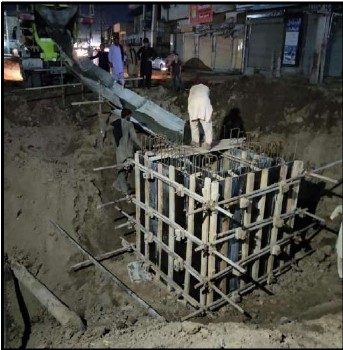
Picture 76: Manhole No. 60 Shaft Concreted at Marala Road
