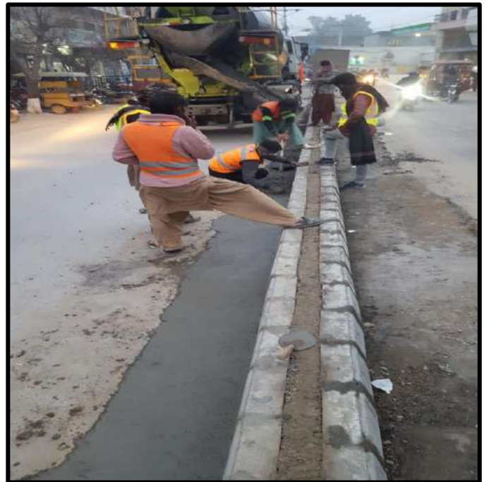
Picture 66: Road Restoration in Progress
