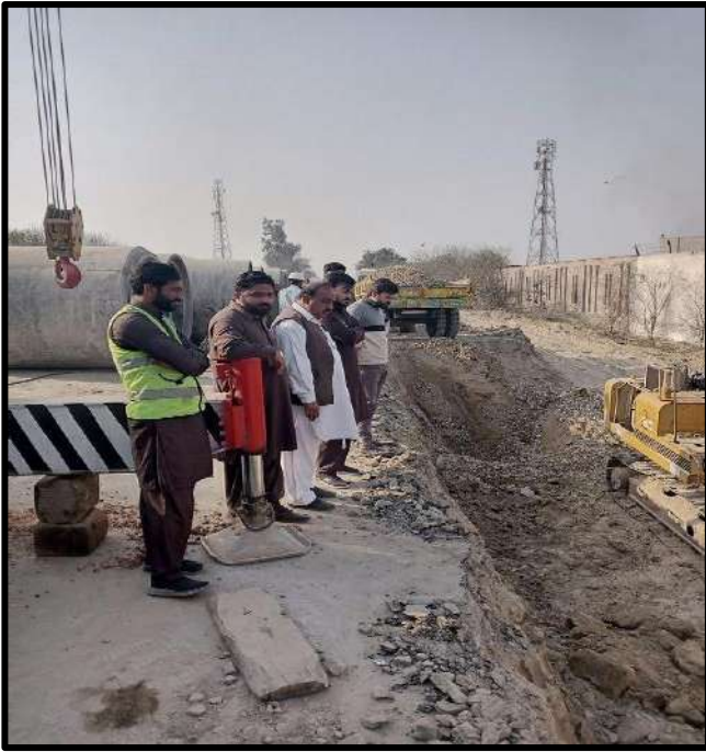
Picture 43: Sewer Bed Preparation
