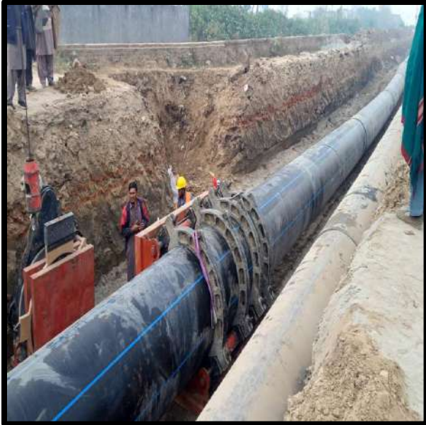
Picture 82: Conduit Placement (Night Shift)
