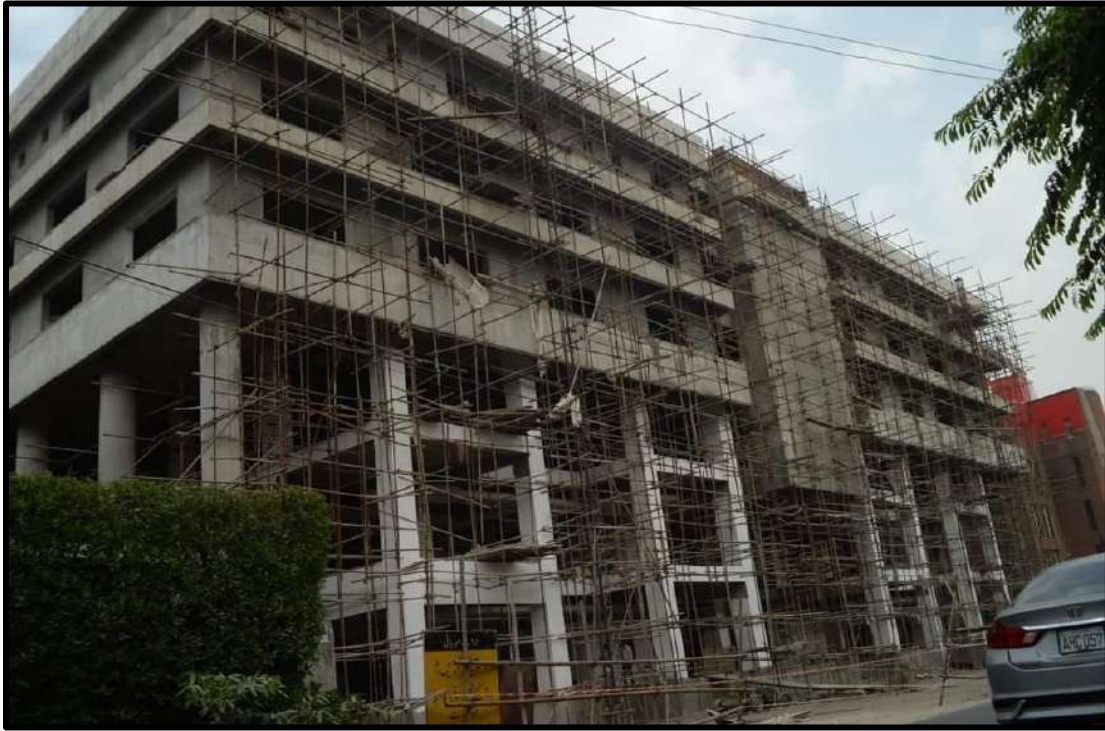
Picture 97: Front Elevation of PLGA Lahore
