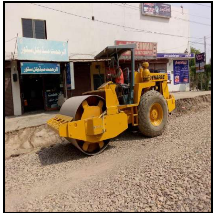
Picture 50: Compaction of WBM In Progress
