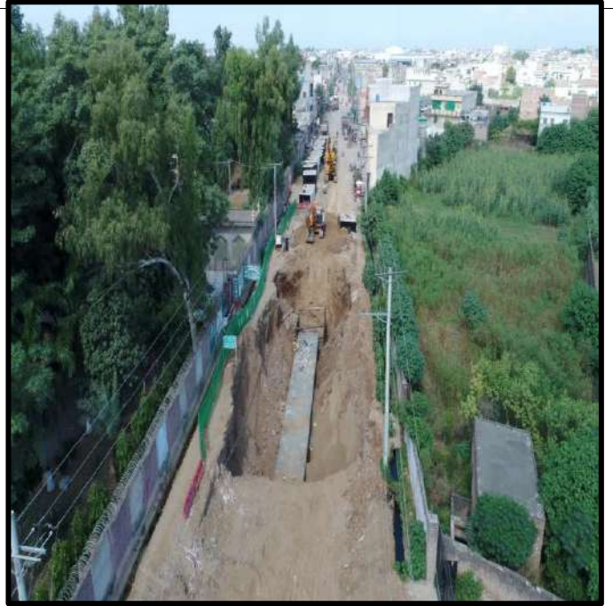
Picture 68: Conduits laying is in progress near Technical College Site 2 Marala Road Sialkot
