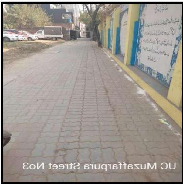
Picture 96: Restoration work at Sialkot
