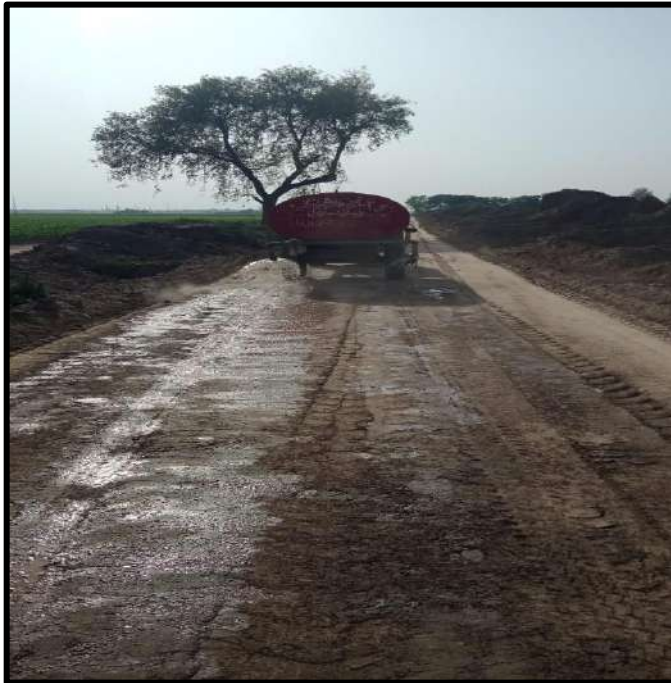
Picture 25: Water Sprinkling is in progress
