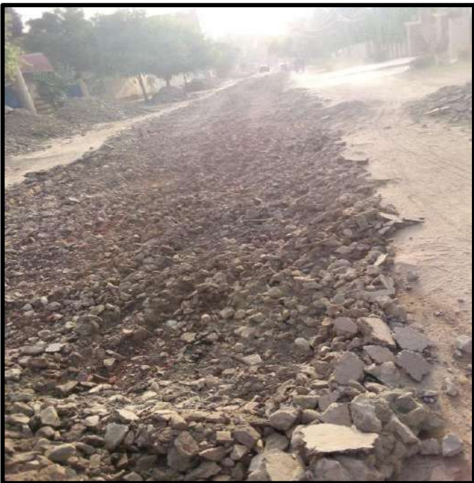
Picture 53: Dismantling at Road-03
