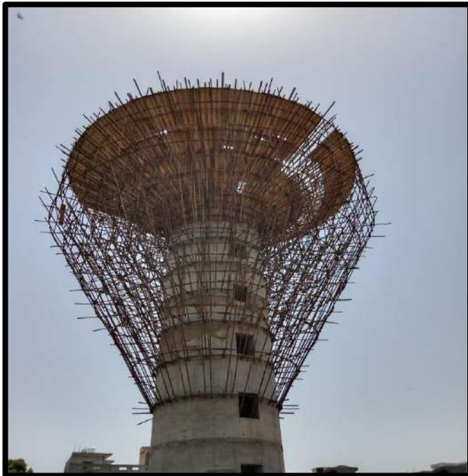
Picture 92: Formwork of Bowl of T-18 Prem Nagar
