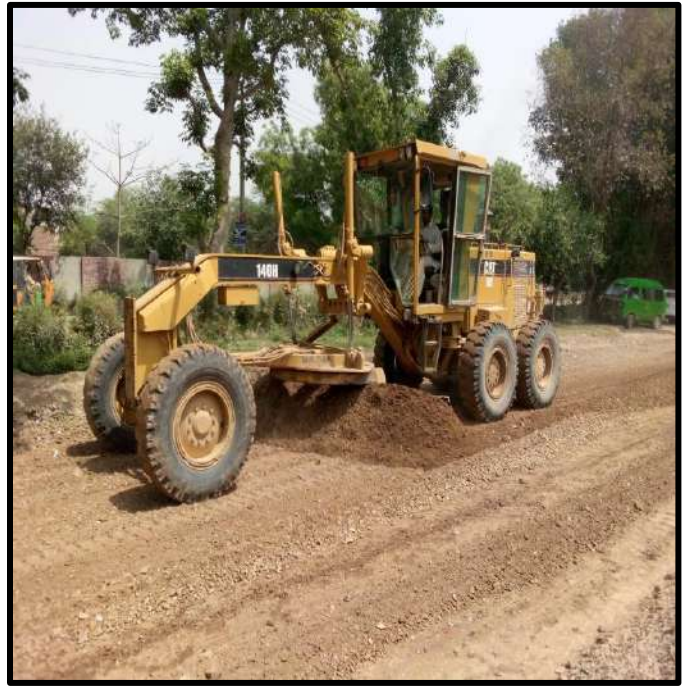
Picture 52: Sub-Base Preparation at Road-03
