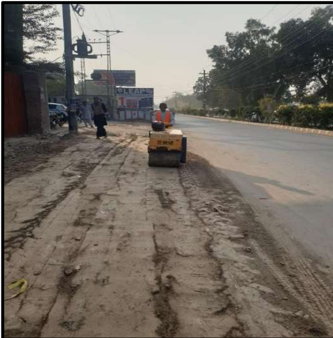
Picture 21: Restoration Work is in Progress
