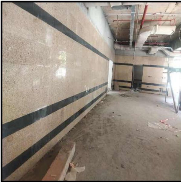
Picture 98: Fixing of Granite on Walls
