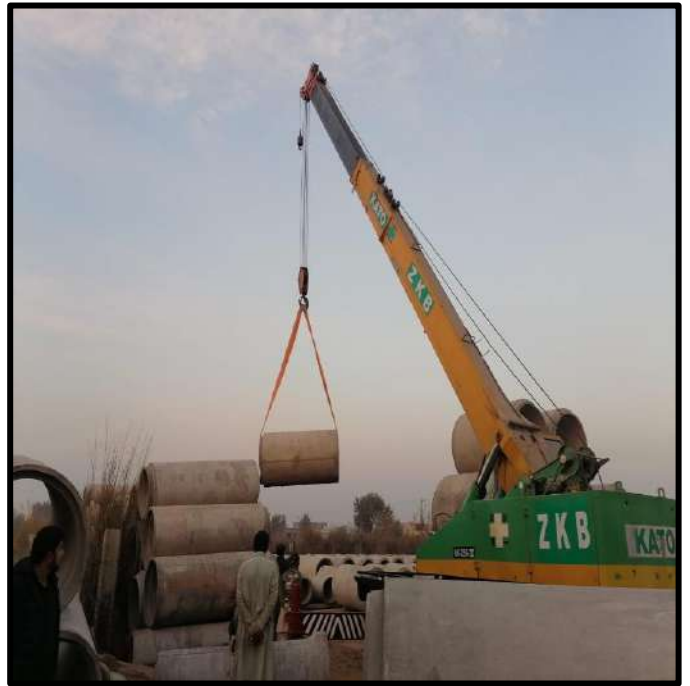
Picture 60: Hauling of Pipe in Progress
