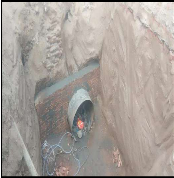
Picture 63: Road Restoration, After Laying of Sewer Line
