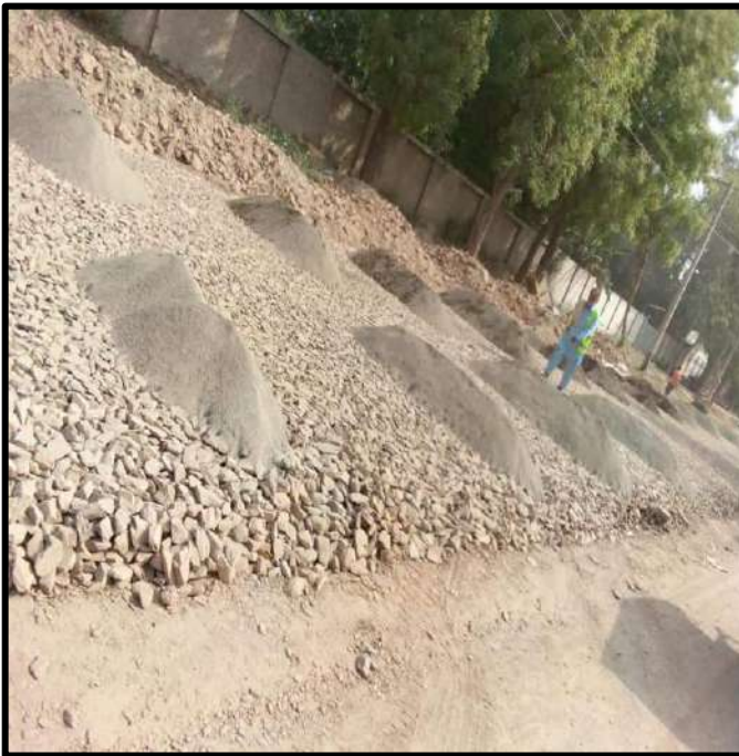
Picture 49: Laying of WBM in Progress
