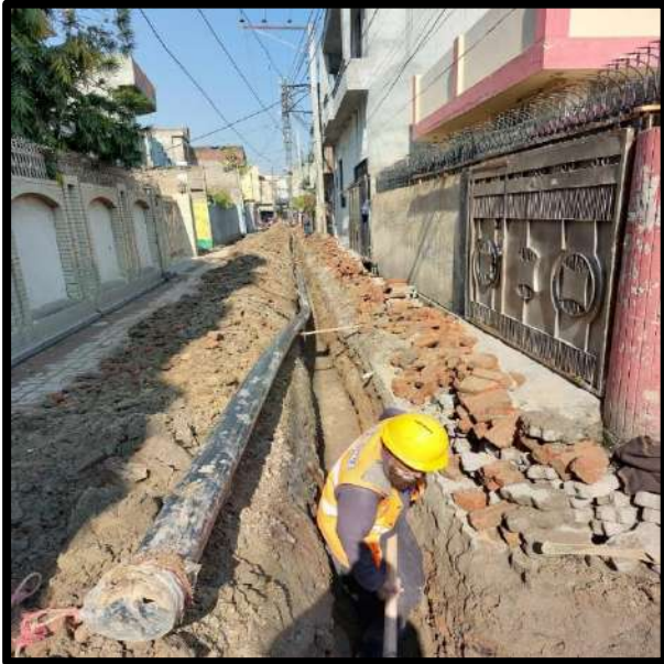
Picture 90: Excavation for Pipe Laying
