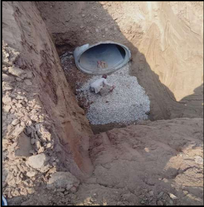
Picture 27: Pipe Laying in Progress
