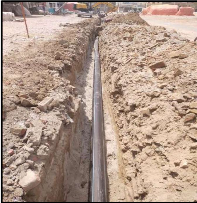
Picture 15: Laying of HDPE pipe is in Progress
