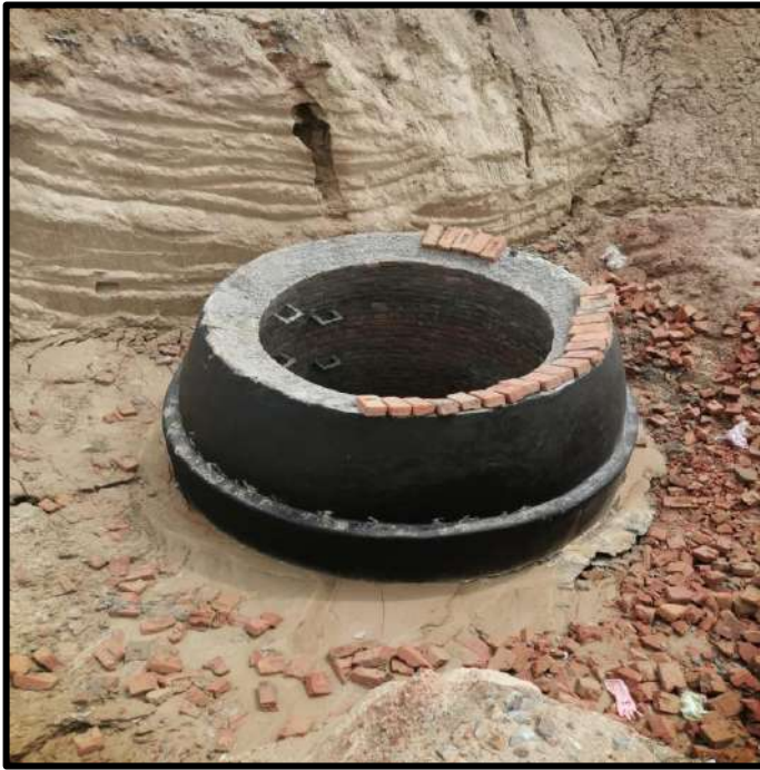
Picture 31: Manhole under Construction
