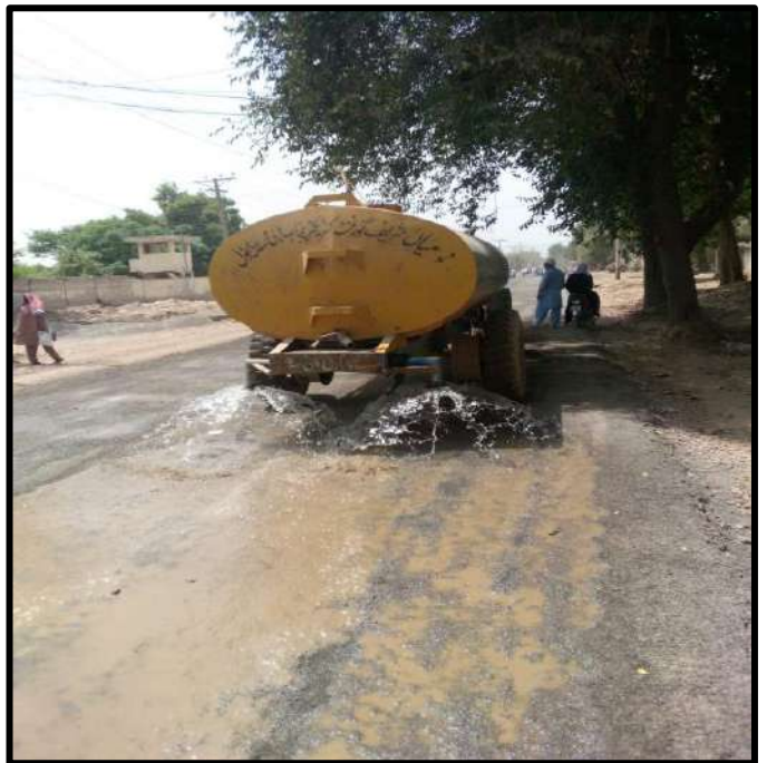
Picture 54: Water Sprinkling at Road 1
