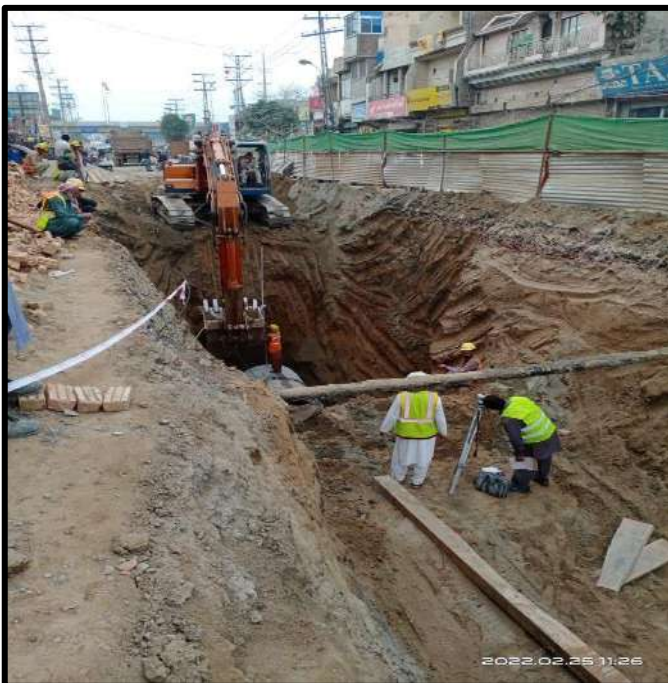
Picture 61: Pipe Laying & Level Inspection in Trench
