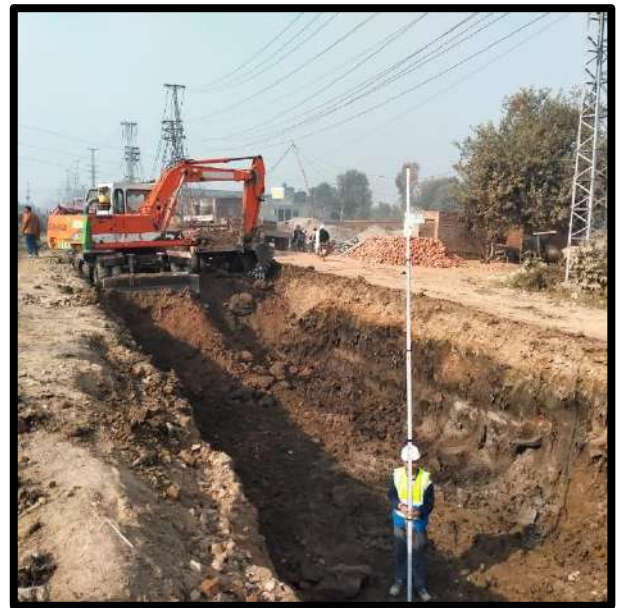
Picture 85: Bed Preparation for layinf of Forcemain
