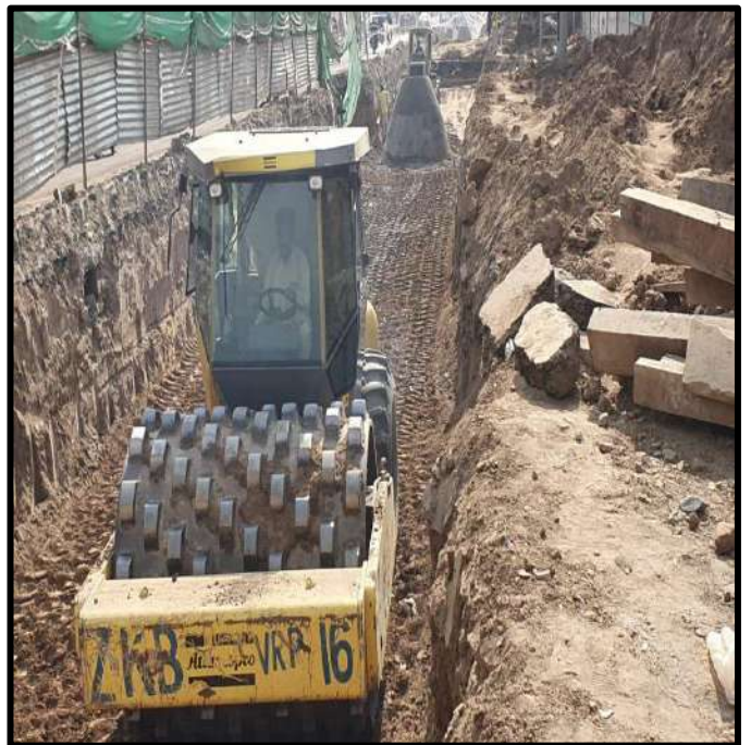
Picture 62: Compaction of Backfill
