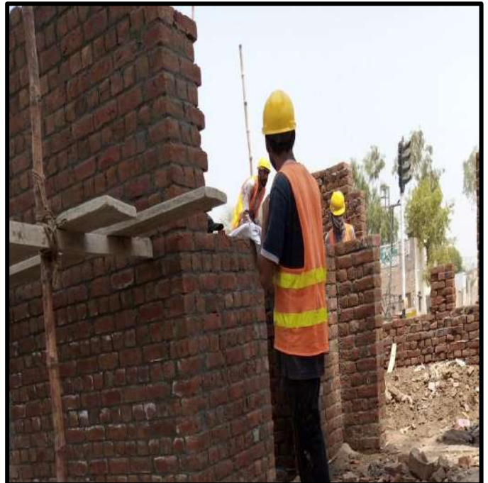
Picture 22: Brick Work at Pump House in progress
