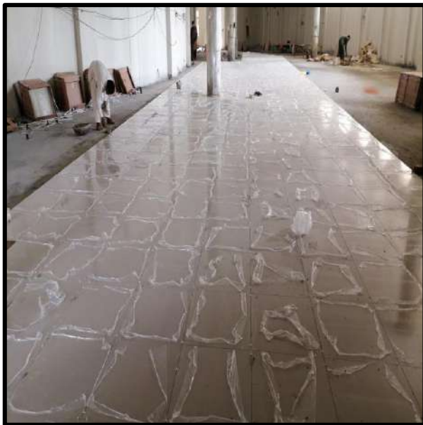
Picture 13: Museum Floor Work at Gulshan-e-Iqbal Park
