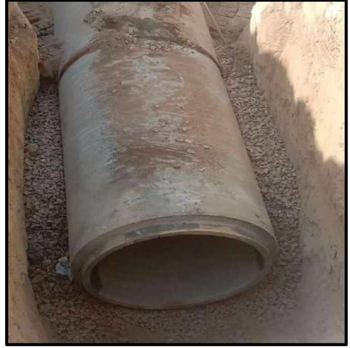
Picture 46: Sewer Laying
