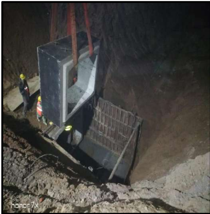
Picture 80: Conduit Placement (Night Shift)
