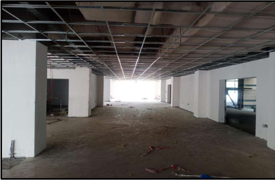
Picture 100: Paint work and fixing of Ceiling Frame
