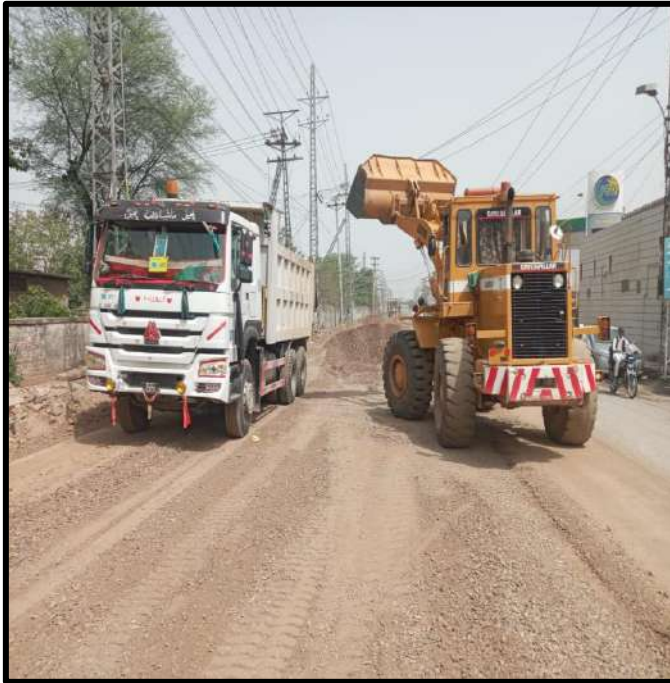
Picture 55: Spreading and Shifting of Aggregate Base Course
