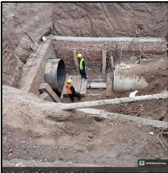
Picture 65: Pipe Laying through Thrust Boring in Progress
