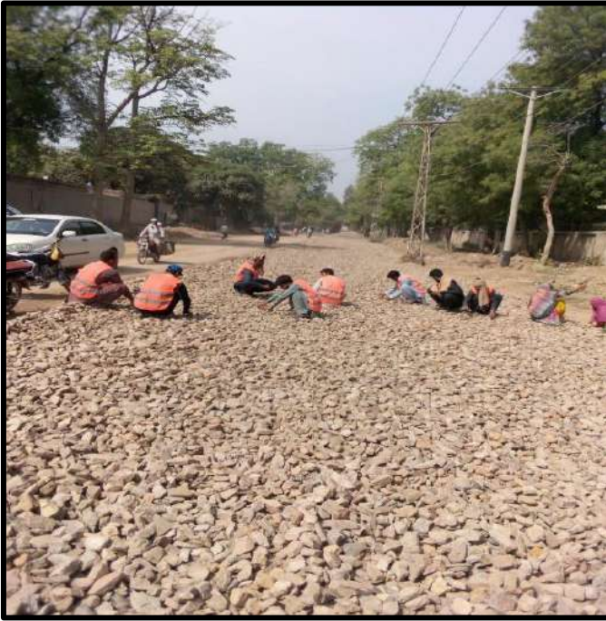
Picture 47: Water Bound Macdum at Fateh Sher Road-01
