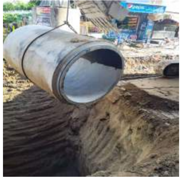
Picture 75: Pipe Laying in Progress
