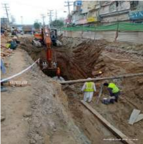
Picture 65: Pipe Laying & Level Inspection in Trench
