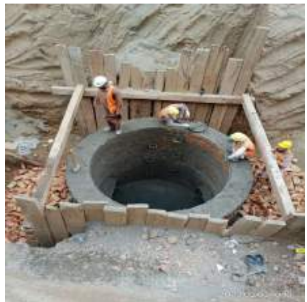
Picture 70: Manhole Construction
