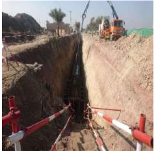
Picture 44: Pouring of Concrete in Progress
