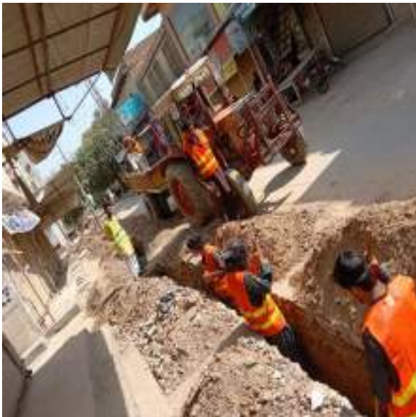
Picture 15: Sand Bedding of Trench AT UC-03
