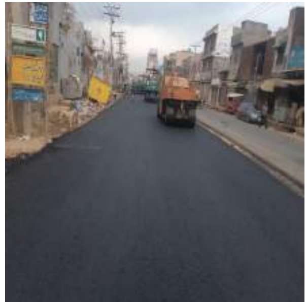
Picture 68: Compaction of Asphalt Concrete Base Course
