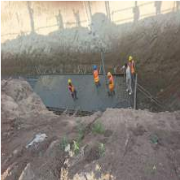
Picture 43: Concrete Roof Slab in Progress, Sahiwal
