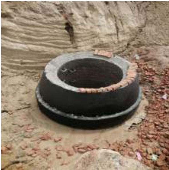
Picture 31: Manhole under Construction
