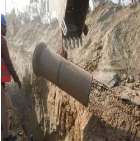
Picture 29: LAYING OF RCC PIPES
