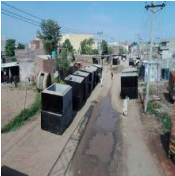
Picture 76: Single Cell Conduits laying is in progress near Sublime Chowk Site 1 Marala Road Sialkot
