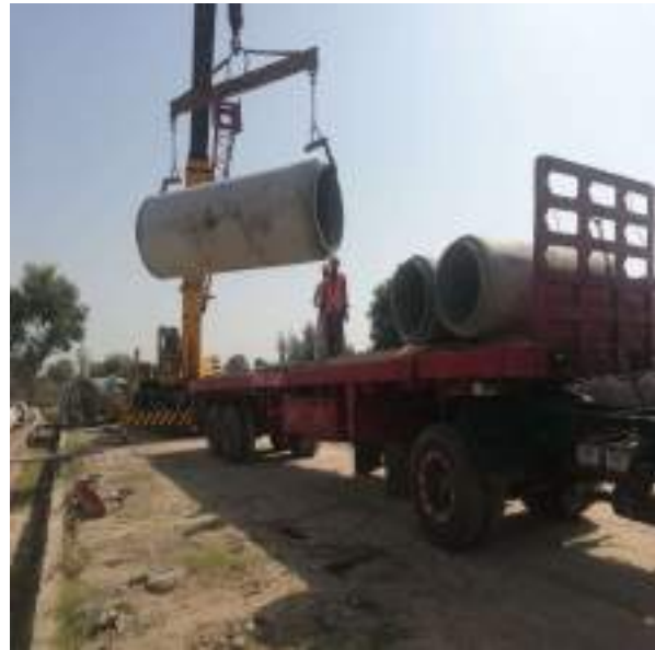
Picture 30: HAULAGE OF RCC PIPES
