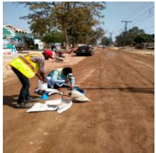
Picture 60: Field Density Test at Road-01
