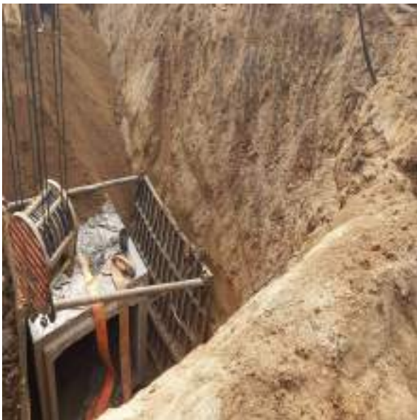
Picture 80: Conduit Placement (Day Shift)
