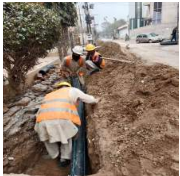
Picture 16: HDPE Pipe laying in Progress
