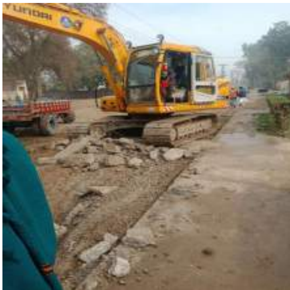
Picture 55: Dismantling of Road-01
