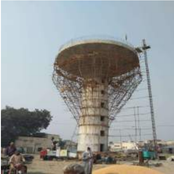
Picture 21: OHR under Construction
