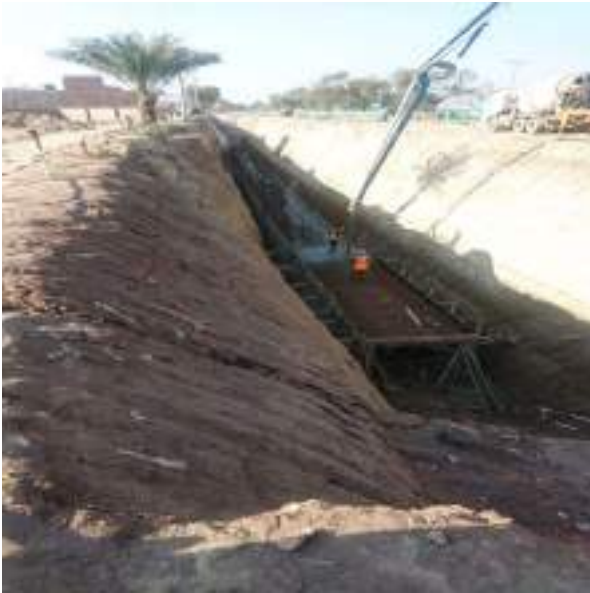
Picture 41: Concrete Roof Slab in Progress, Sahiwal
