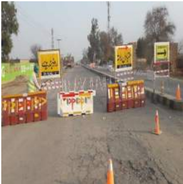
Picture 47: Work in progress and Diversion provided
