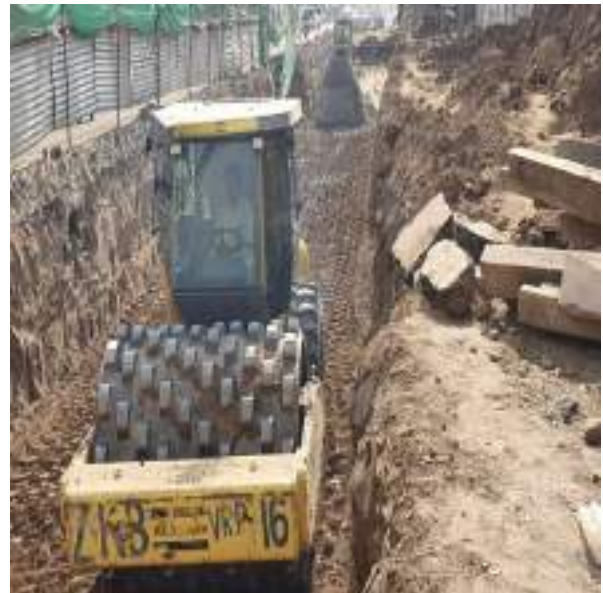
Picture 66: Compaction of Backfill
