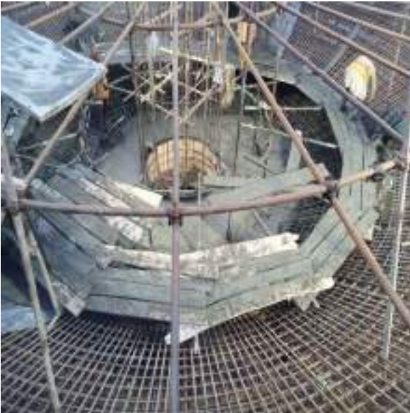
Picture 96: Construction of OHR in Progress
