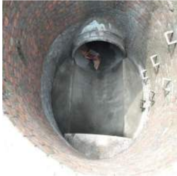
Picture 36: Manhole Benching completed Lot-02
