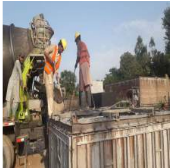
Picture 85: Conduit Manufacturing in Process
