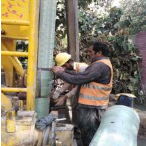
Picture 17: Pipe Lowering of Tube well
