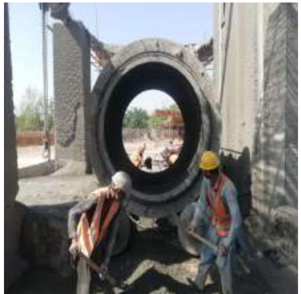
Picture 24: Manufacturing of RCC Pipe
