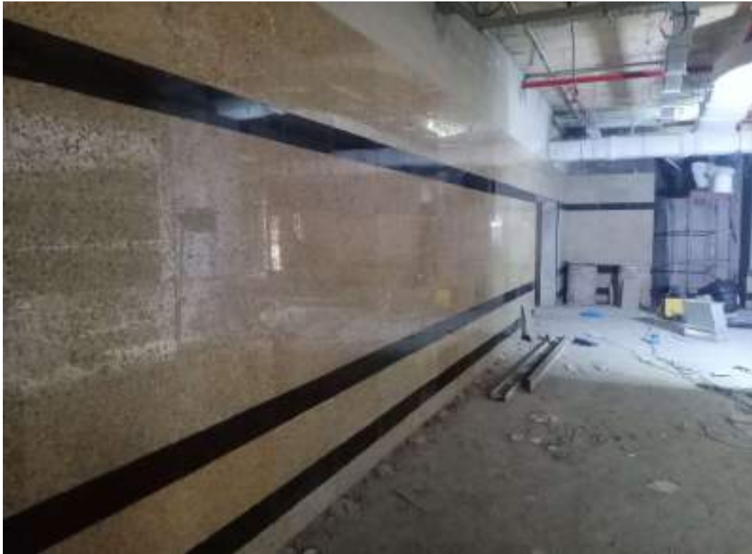
Picture 104: Project Progress View of Internal Side Wall dated 28.02.2022
