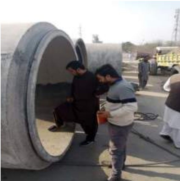
Picture 51: Sewer Checking at Factory
