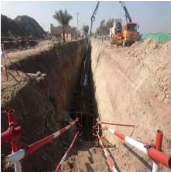
Picture 39: Acces to the Conduit which is in Progress
