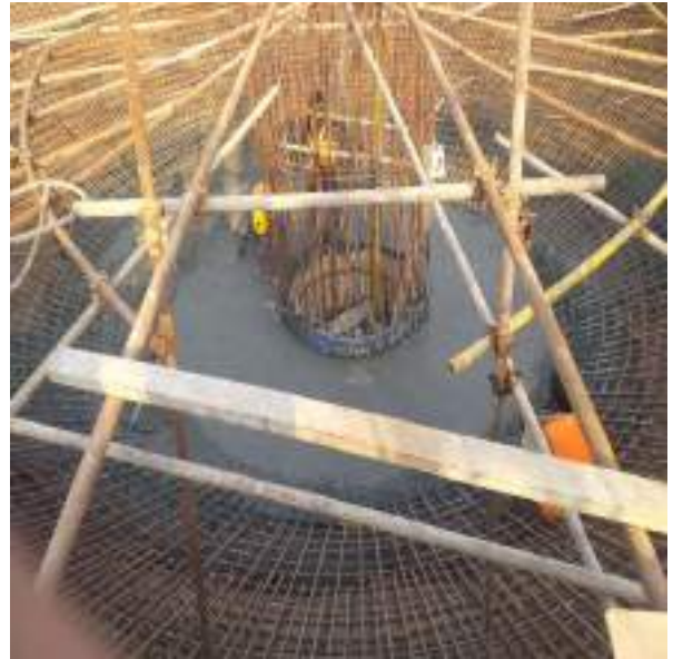
Picture 22: Bowl Concrete Pouring T#7 Ghalla Mandi
