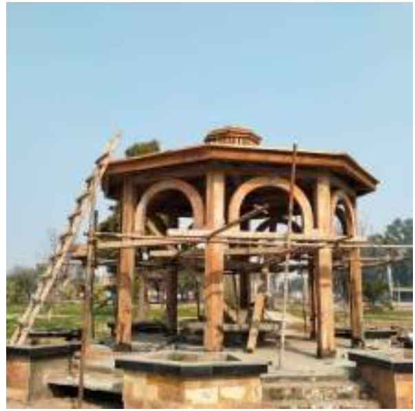
Picture 8: Gazebo wood work in Progress at Gulshan-e-Iqbal Park
