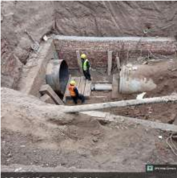
Picture 72: Pipe Laying through Thrust Boring in Process
