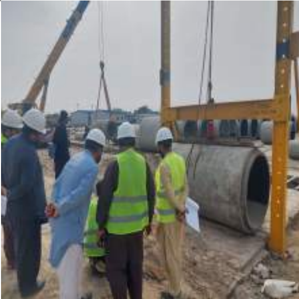
Picture 49: Brickwork of Manhole
