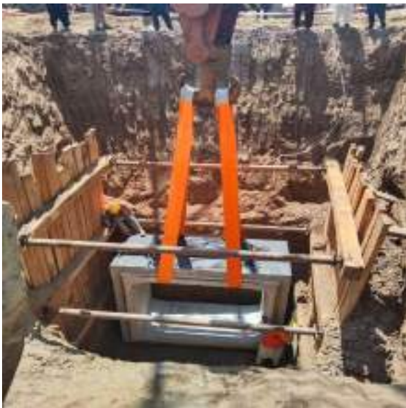
Picture 84: Conduit Placement in Process
