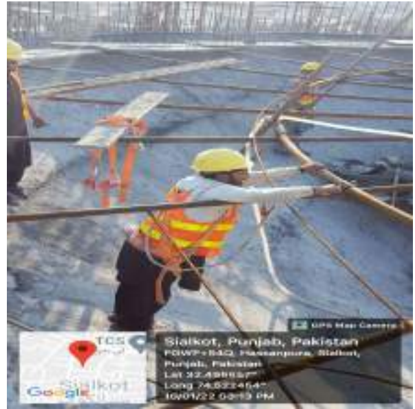
Picture 95: Shuttering Arrangement for OHR
