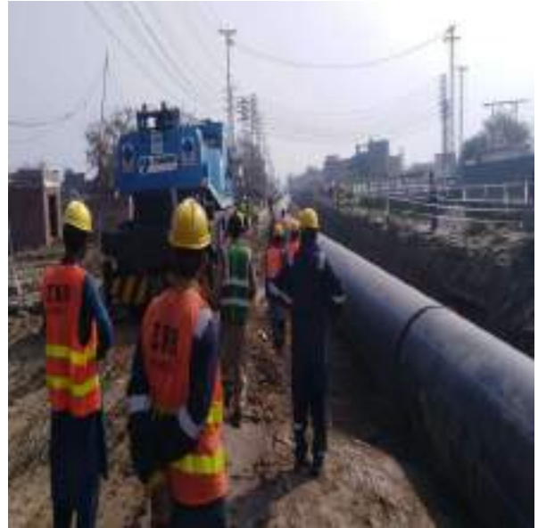
Picture 87: Backfill Restoration
