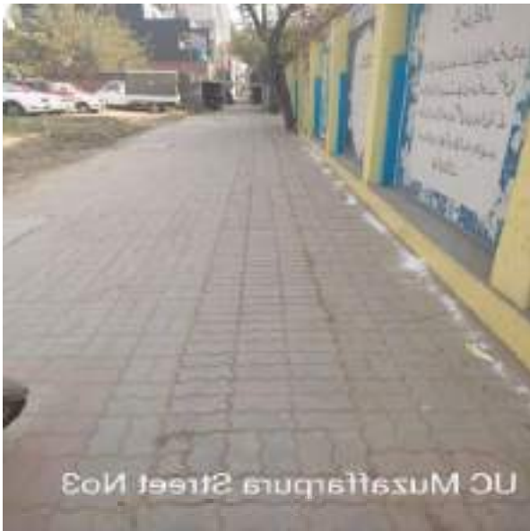
Picture 100: Restoration work at Sialkot
