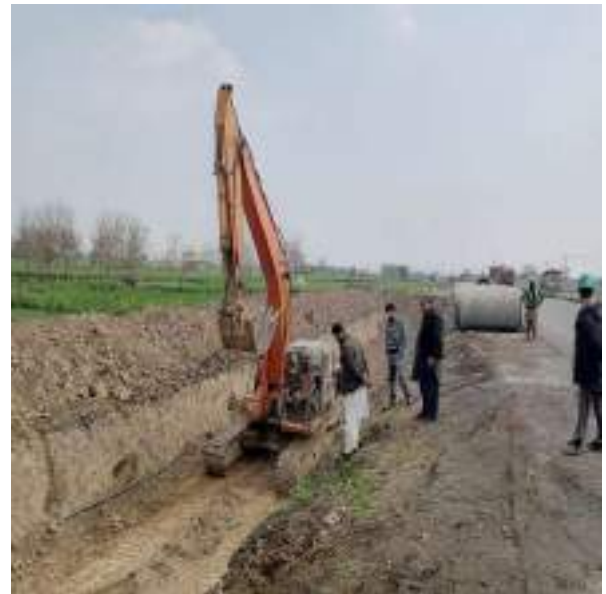
Picture 48: Sewer Bed preparation
