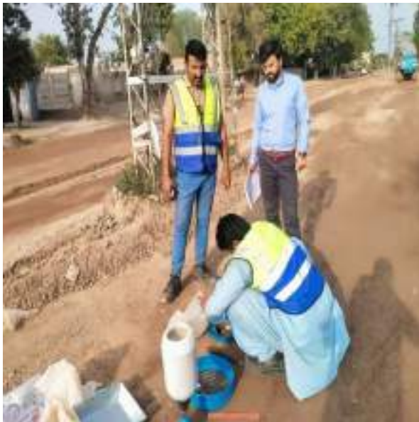
Picture 59: Field Density Test at Road-01
