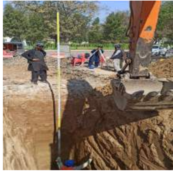
Picture 28: Manhole under Construction
