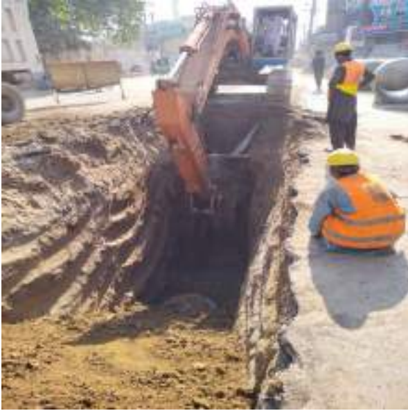
Picture 74: Pipe Laying in Progress
