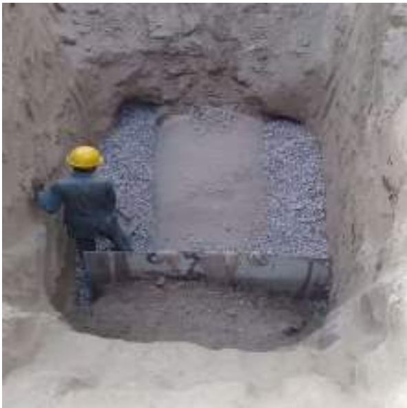
Picture 35: Pipe Bedding with Hunching Lot-02
