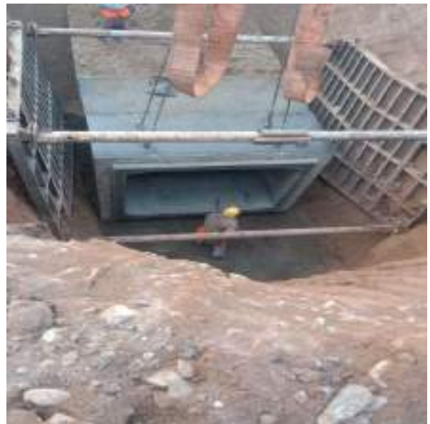
Picture 81: Conduit Laying
