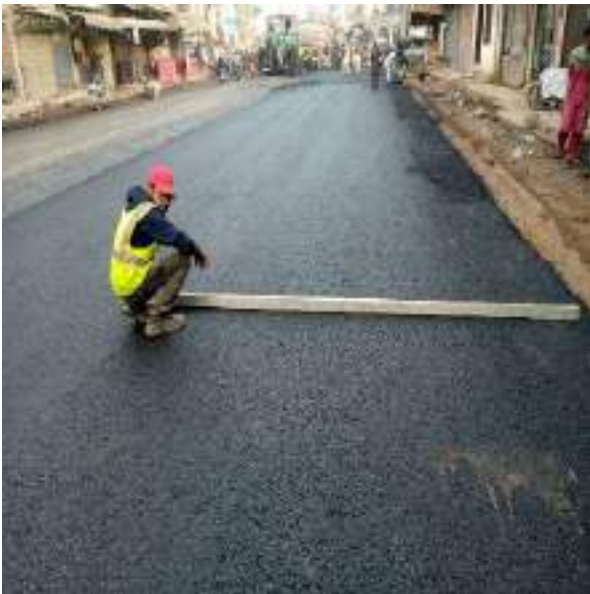
Picture 69: Inspection of Laid Asphalt Grade with Straight Edge
