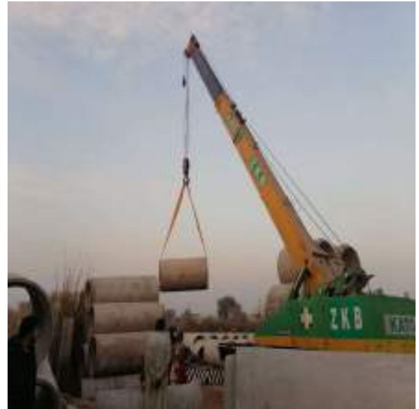
Picture 64: Hauling of Pipe in Progress
