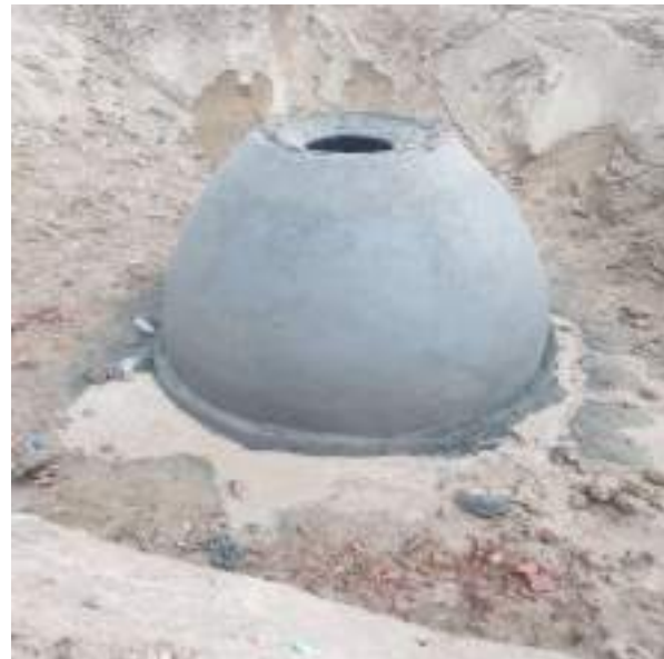
Picture 32: Manhole under Construction
