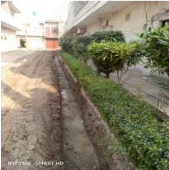
Picture 13: Watering Ramming at Water Supply Lot-01
