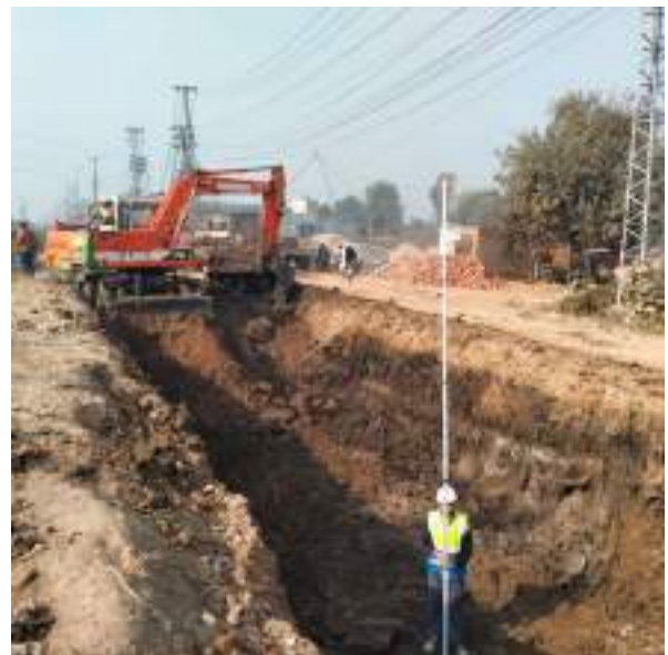
Picture 89: Bed Preparation for layinf of Forcemain
