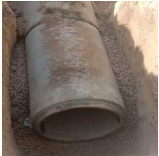
Picture 52: Sewer Laying
