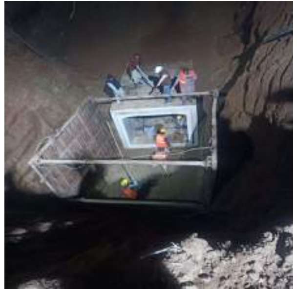
Picture 83: Backfill Restoration
