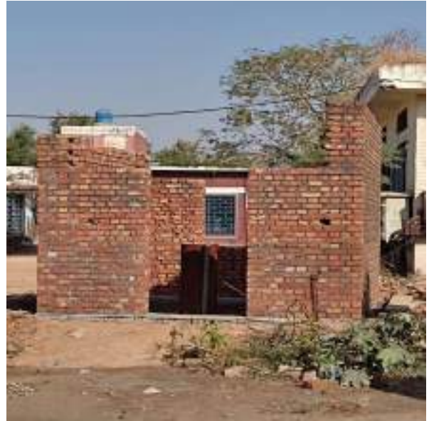
Picture 91: Brick work of Pump Room in Mayana Pura
