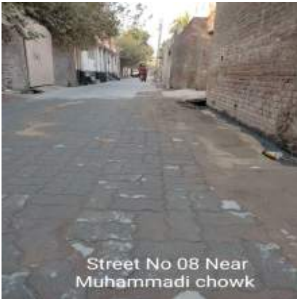
Picture 92: RESTORATION WORKS PICTURES OF LOT-04
