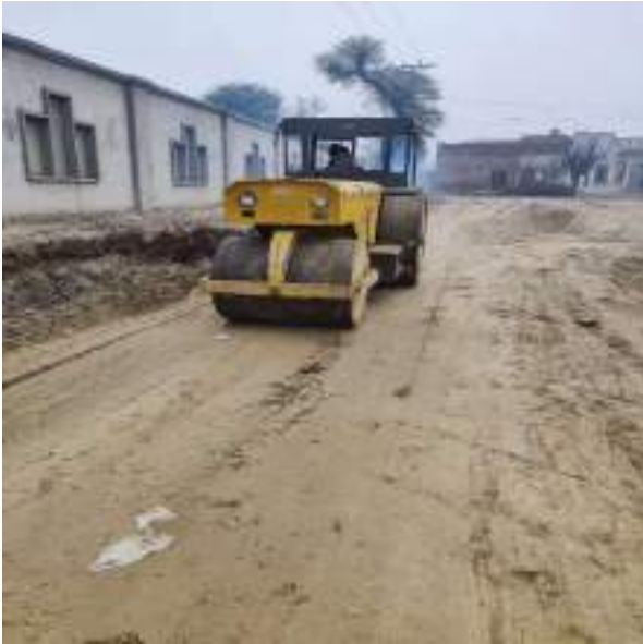
Picture 53: Compaction of Road after Laying of Sewer Line
