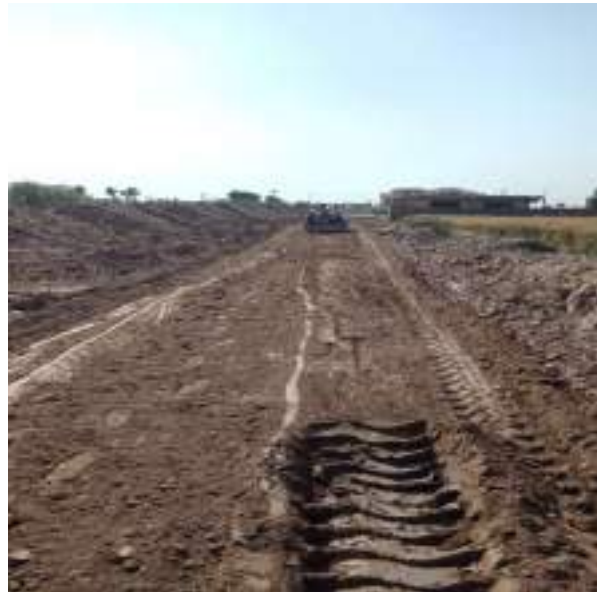
Picture 34: Compaction work is in Progress
