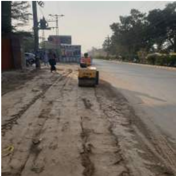
Picture 19: Restoration Work is in Progress
