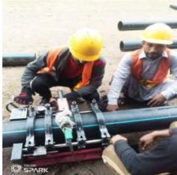
Picture 18: HDPE Pipe Jointing At UC-10
