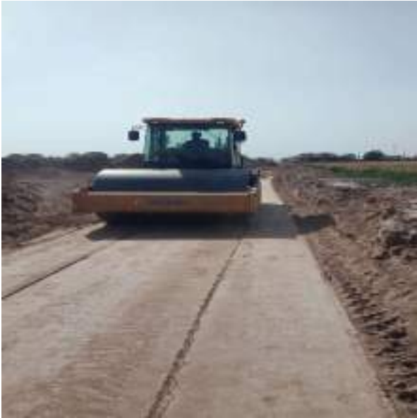
Picture 33: Compaction work is in Progress
