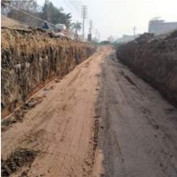
Picture 90: Sewer Bed Preparation
