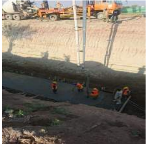
Picture 42: Concrete Roof Slab in Progress, Sahiwal
