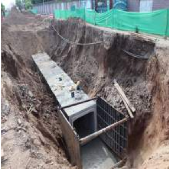
Picture 78: Conduits laying is in progress near Technical College Site 2 Marala Road Sialkot
