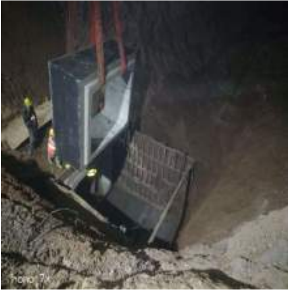
Picture 82: Conduit Placement (Night Shift)
