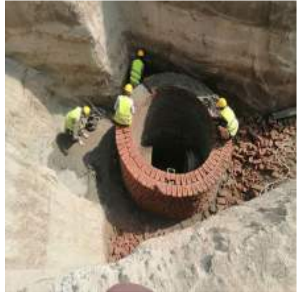
Picture 46: Manhole under Construction
