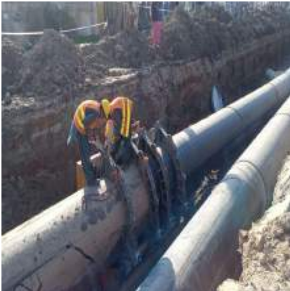
Picture 88: Welding of Forcemain
