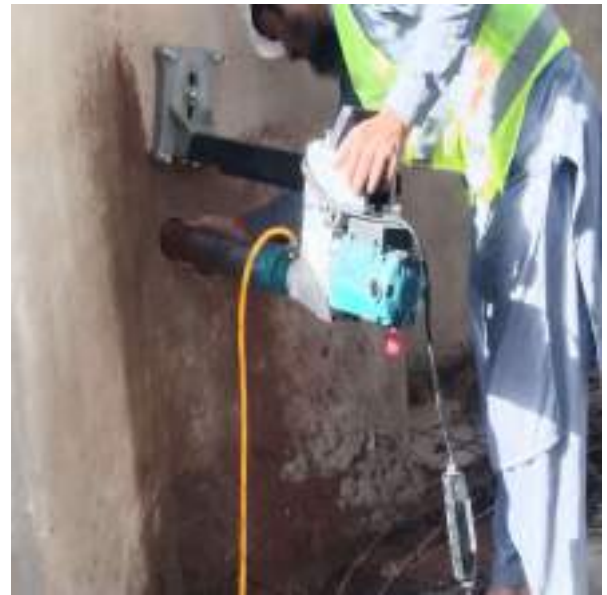
Picture 14: Core Cutting of OHR for Rehabilitation purpose
