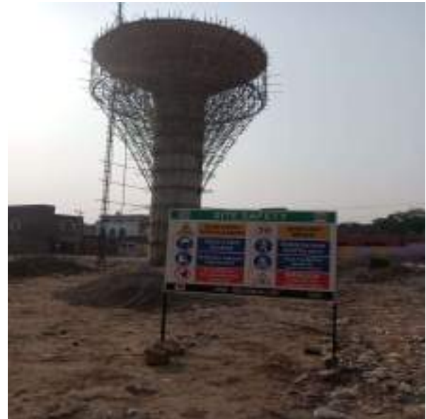
Picture 97: Construction of OHR in Progress
