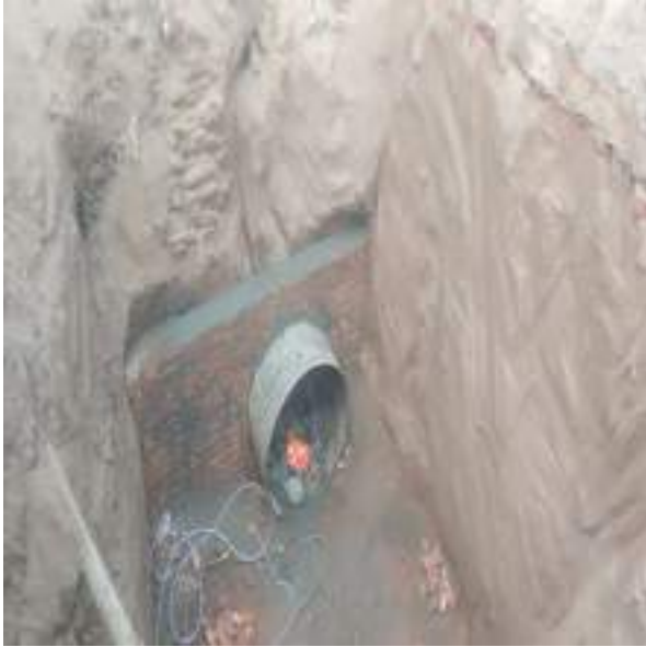
Picture 67: Pipe Laid and backfilled
