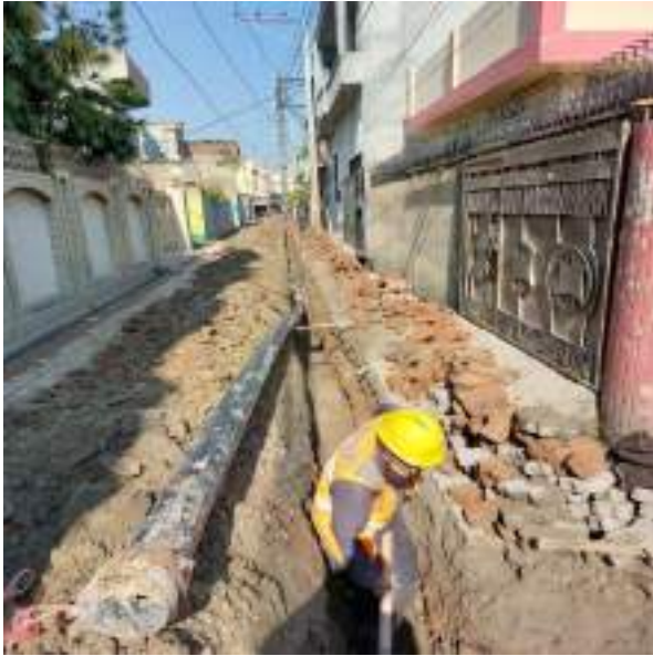
Picture 94: Excavation for Pipe Laying
