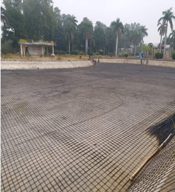
Picture 10: Flooring work of Gazebo at Abdul Hakeem Park
