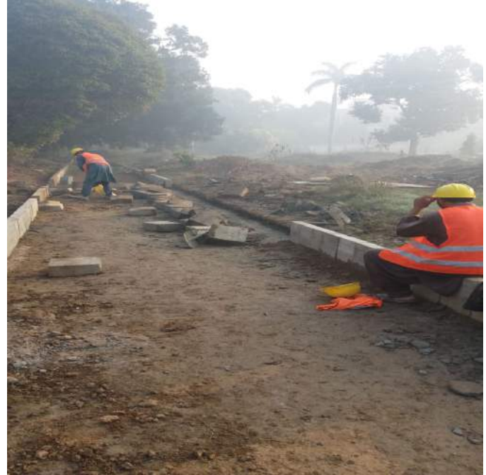
Picture 15: Construction of Jogging Track at Gulshan-e-Iqbal Park
