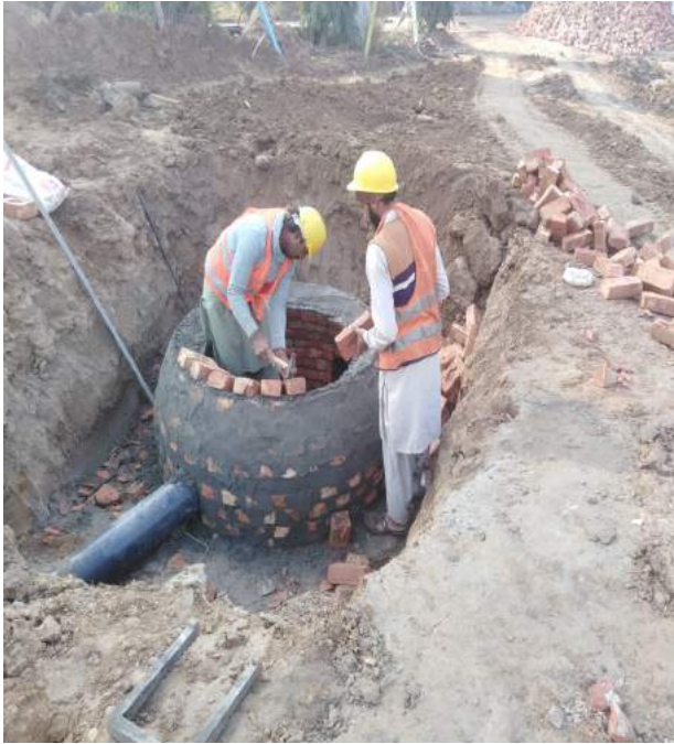
Picture 14: Construction of Sewer Manhole at Gulshan-e-Iqbal Park
