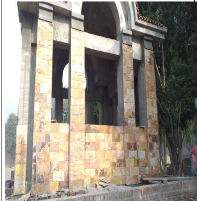
Picture 7: Fixing of Natural Stone on Kiosk at Chaman Zar Park
