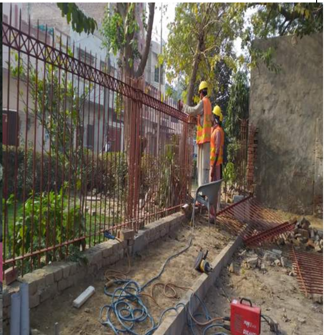
Picture 8: Fixing of Boundary Wall Grill, Chaman Zar Par
