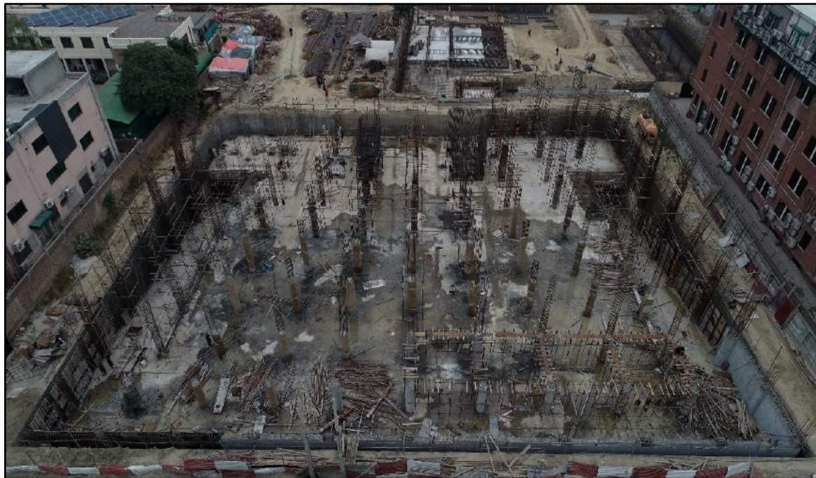
Picture 25: Steel Fixing & Concreting of Basement – 1 Columns
