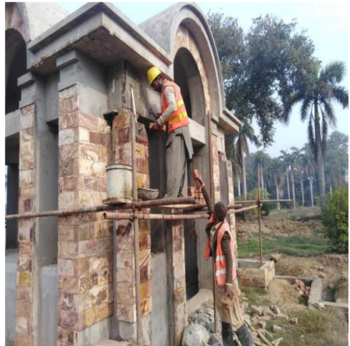
Picture 13: Ceramic Tiles Fixing in Toilet Block of Abdul Hakeem Park
