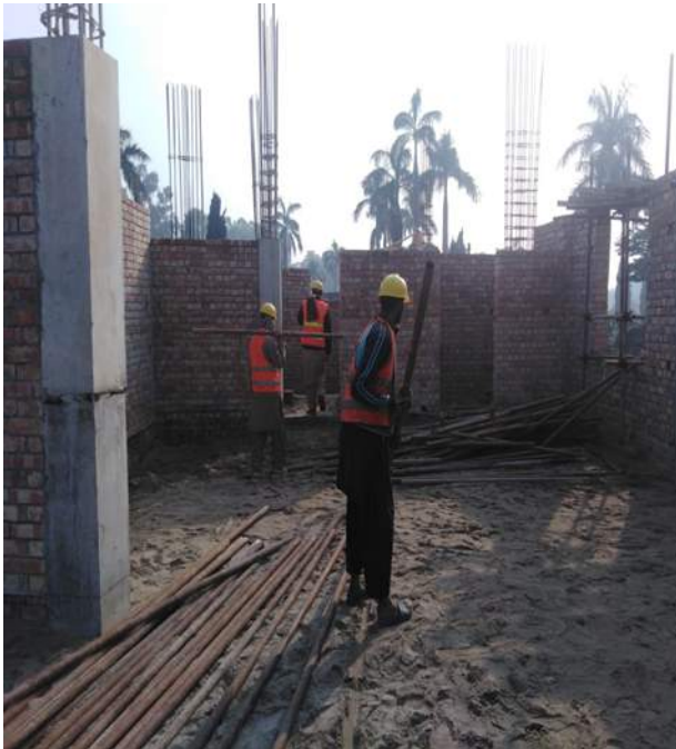
Picture 12: Plinth Protection work of Kiosk at Sialkot Fort Park
