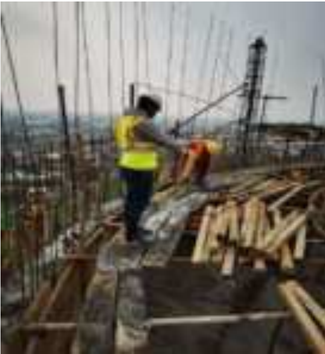
OHR Roof Concreting
