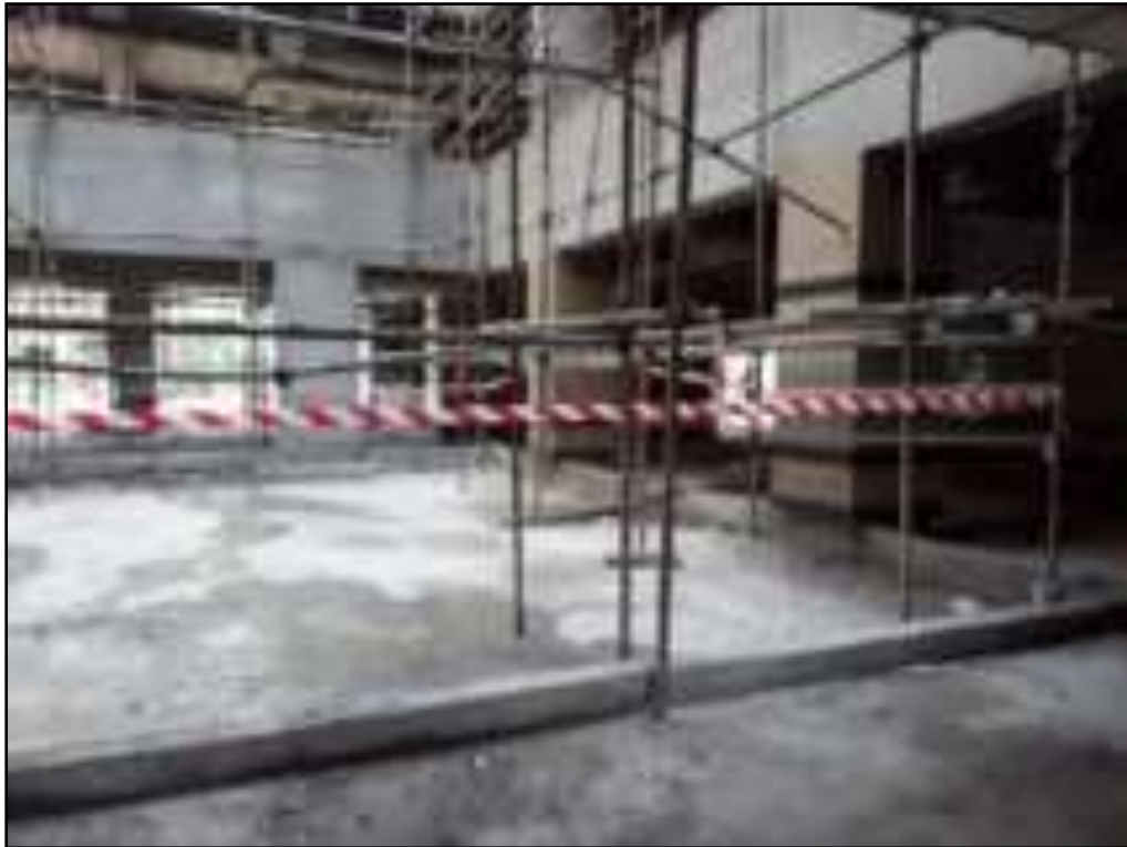
Proper Housekeeping on site
