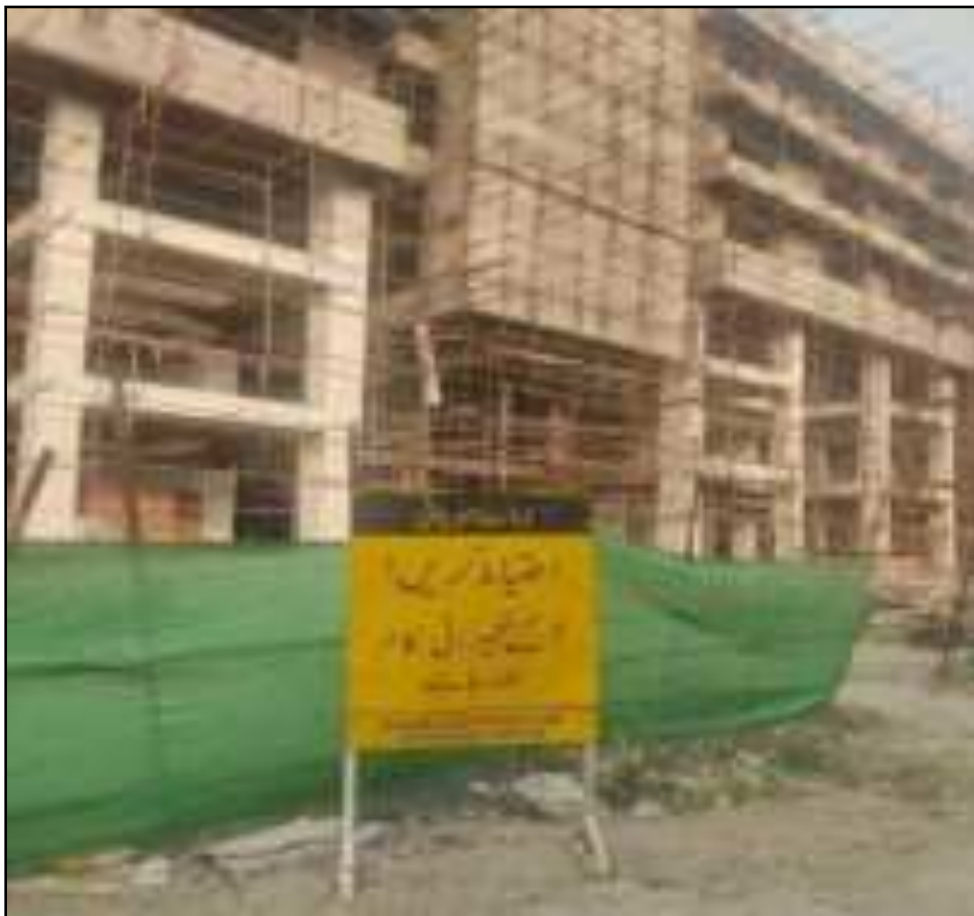
Safety signboard on entrance dated 25-09-2022
