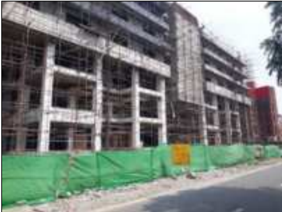
barrication sheet with hard railing and safety signboard
