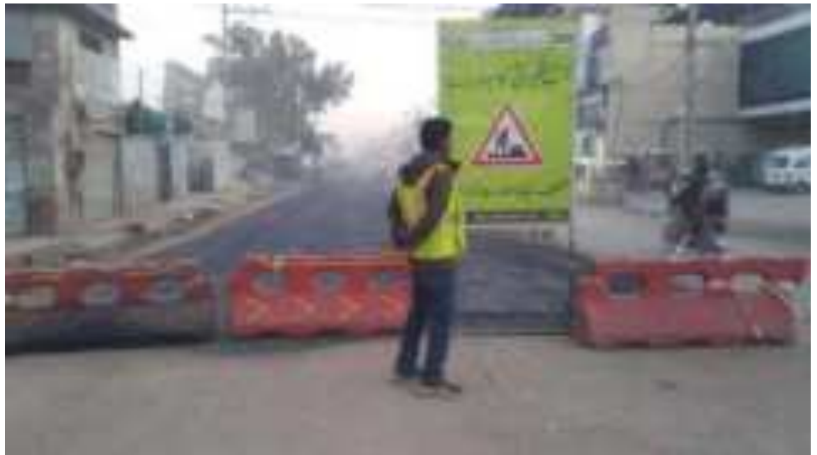
Safety Signs and Barriers and hard Barricade
