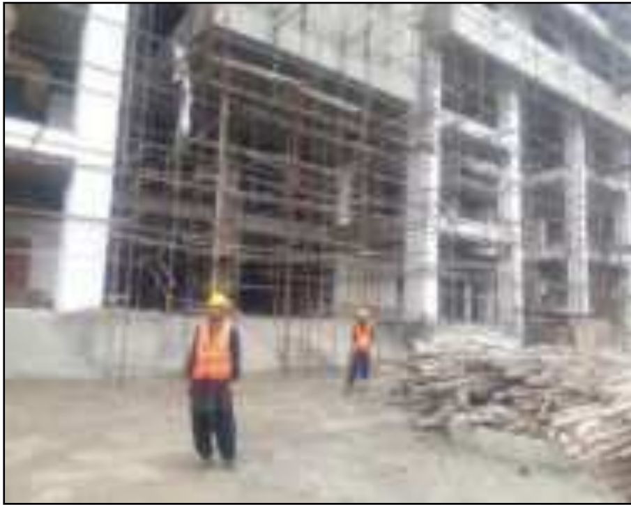
Proper housekeeping and stacking of folding pipes
