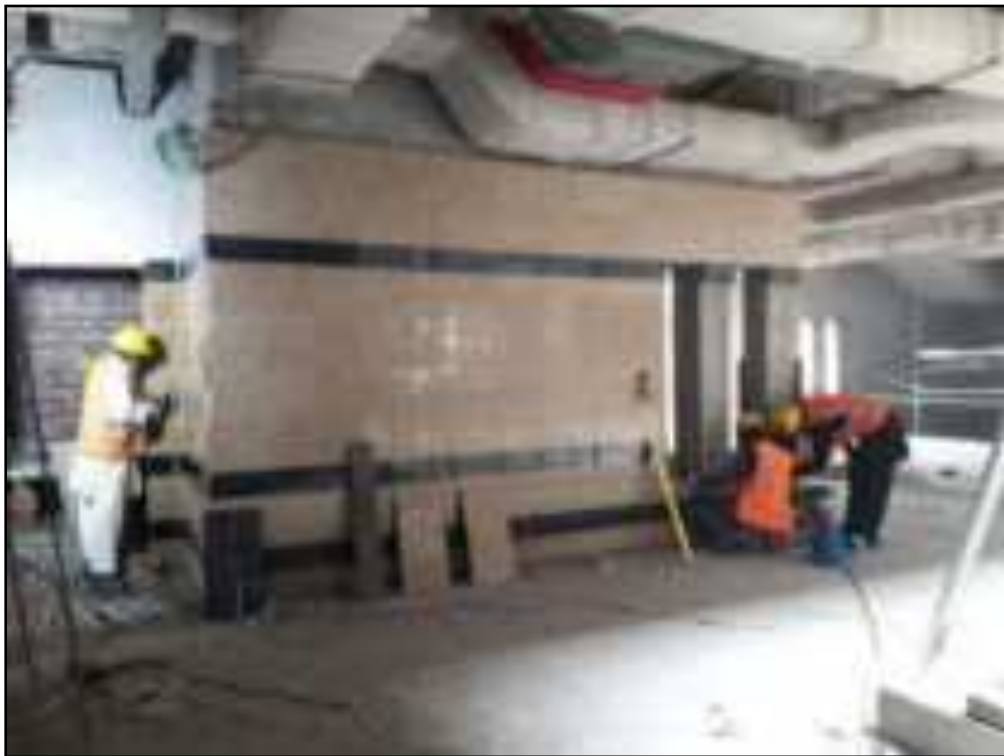
use of PPES on site
