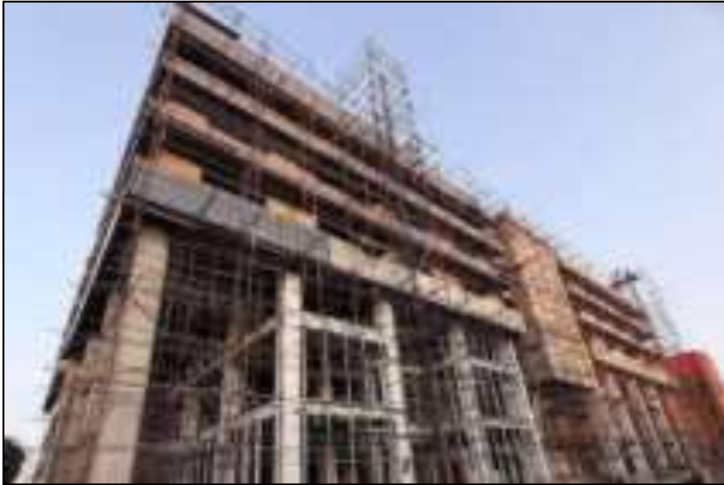
Site work progress
