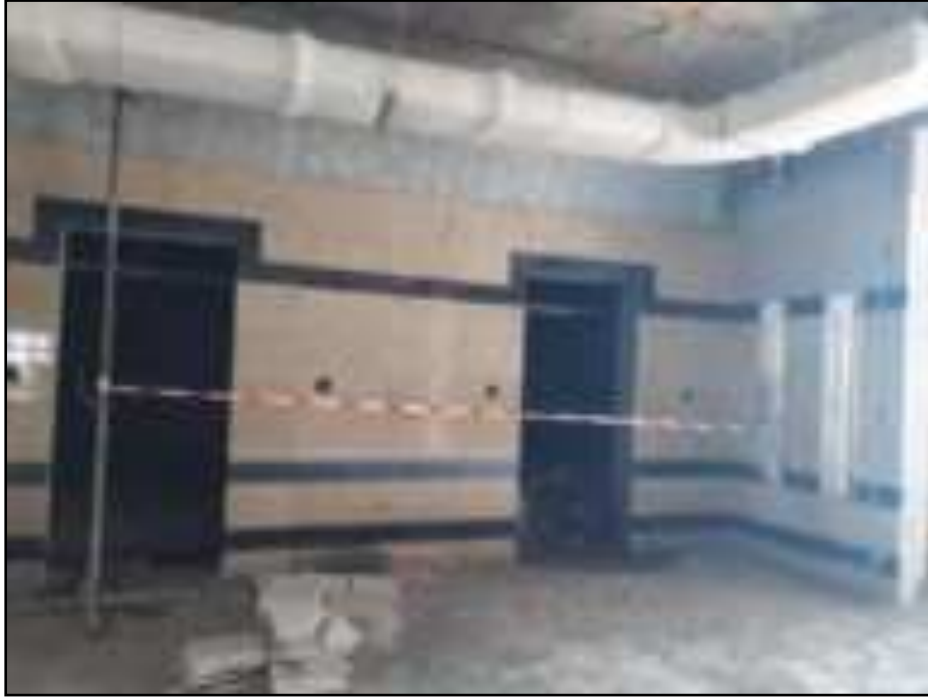
Figure: B Barricade on elevators gate
