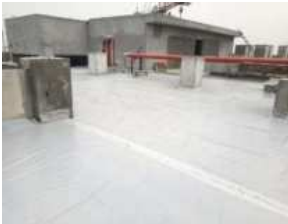
Bitumen Coating and Polythene Sheet at Roof
