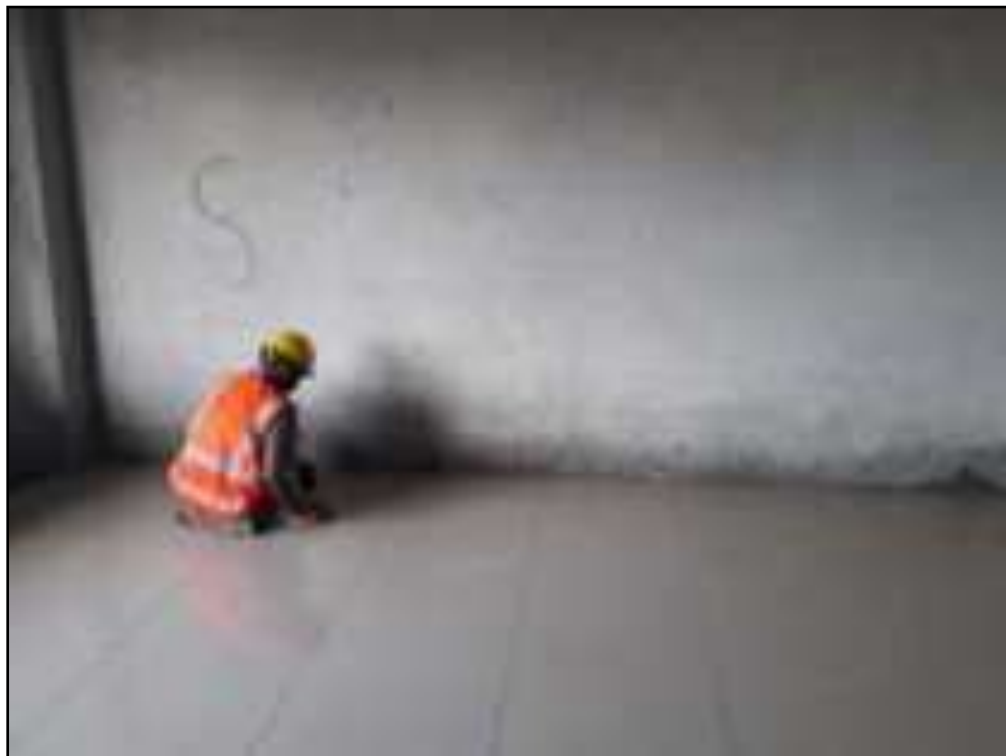
Tile work with use of PPes
