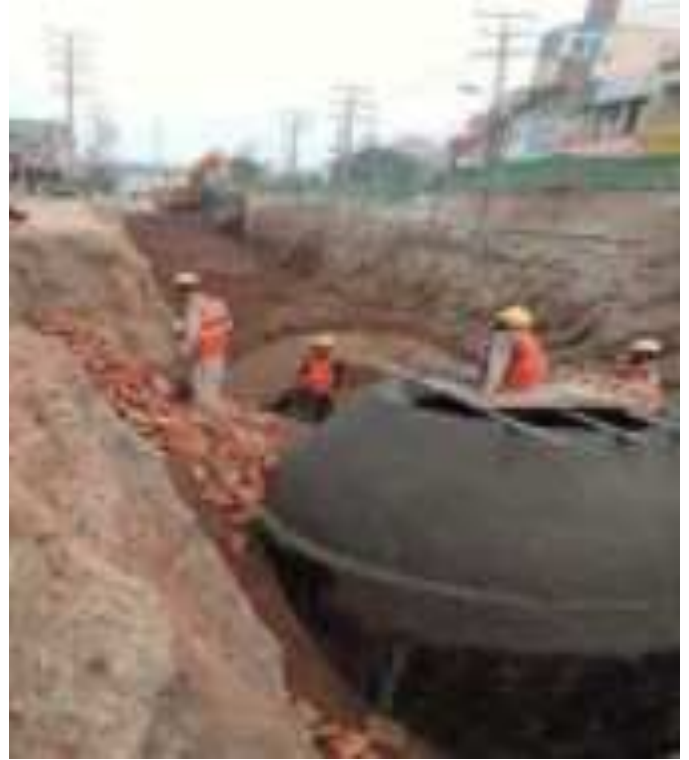
Manhole Construction in Progress
