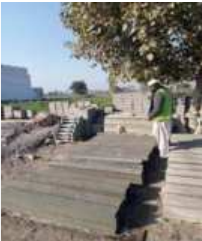
Boundary Wall Fence Post Curing & Self-Inspection
