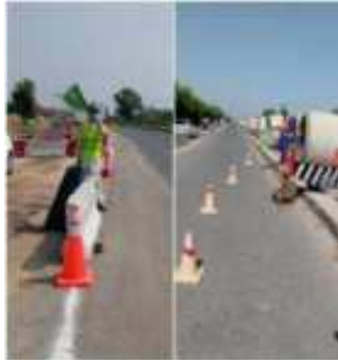
Flagman's are deployed at diversion route to the control traffic
