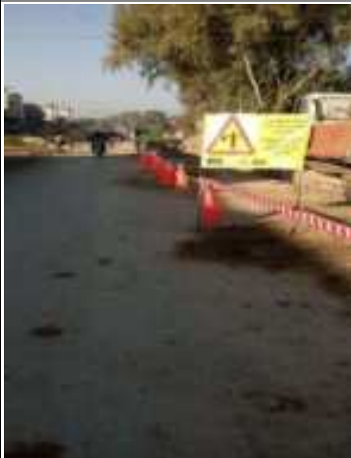
Safety sign board and Safety cones are placed on Road for public awareness
