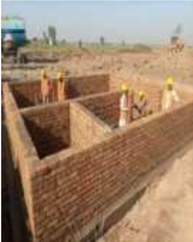
Committed Work with Complete PPEs
