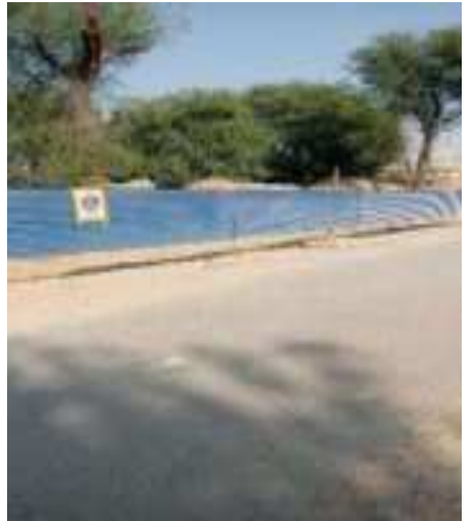
Hard barricading installed near deep excavation trench at different project sites.
