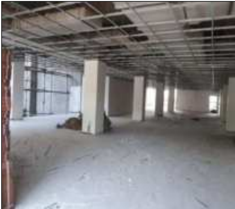
Site Ceiling work progress
