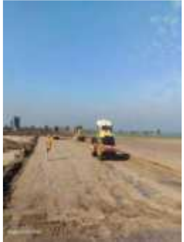
Site Work in Smooth Way
