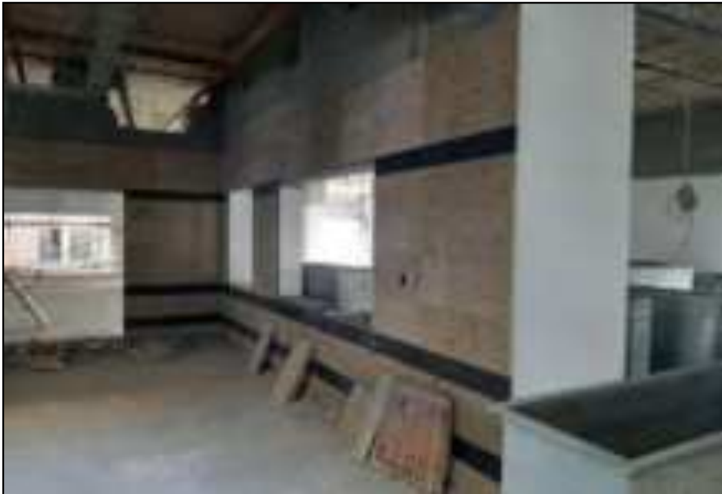
Marble Work progress
