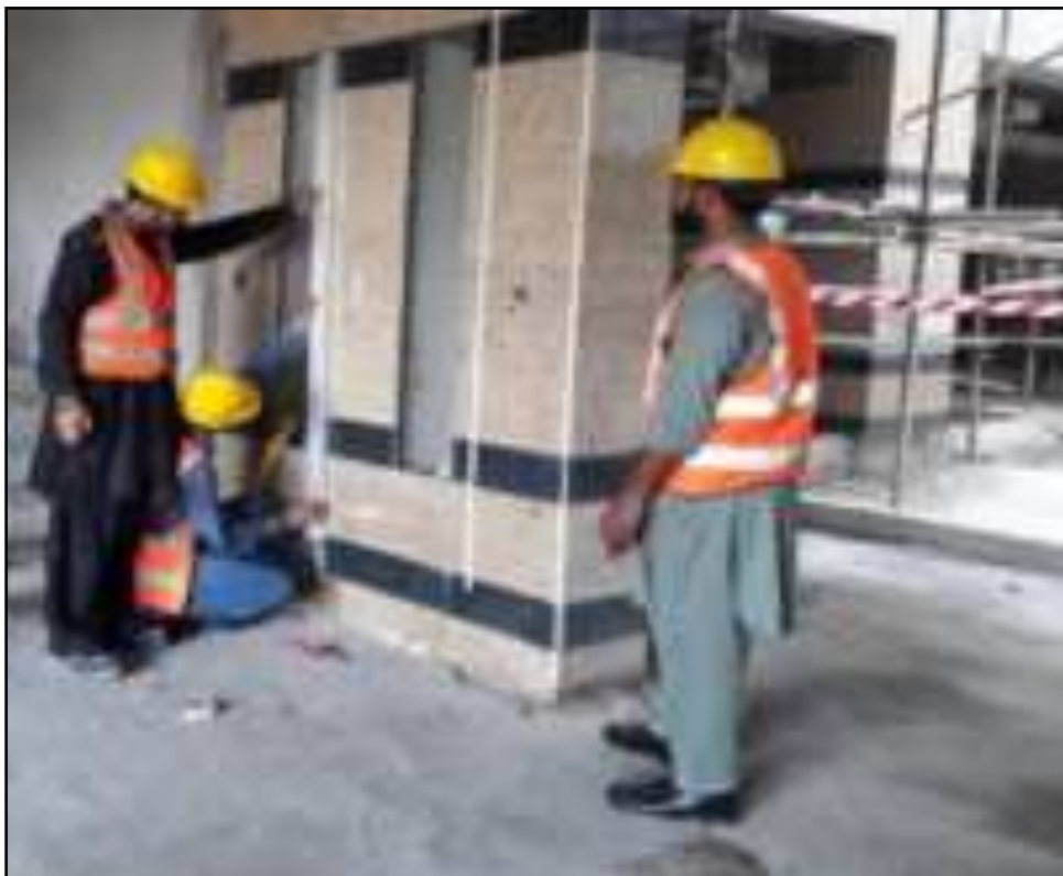
Use of PPEs during work
