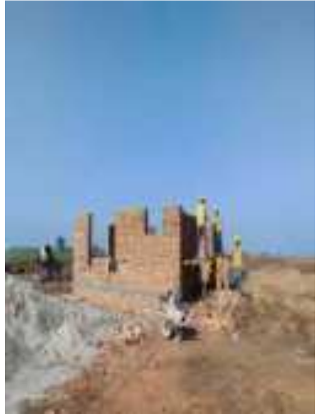
Building Works in Progress
