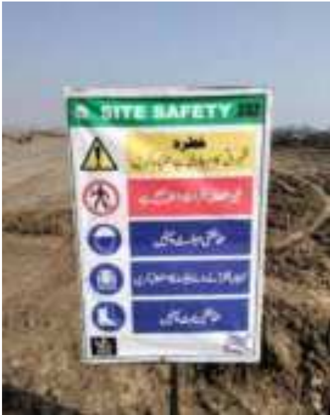
Informatory Safety Sign Board of "Site Safety" on-site
