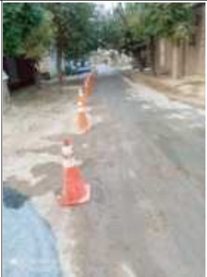
Safety cones are placed on Road for public awareness
