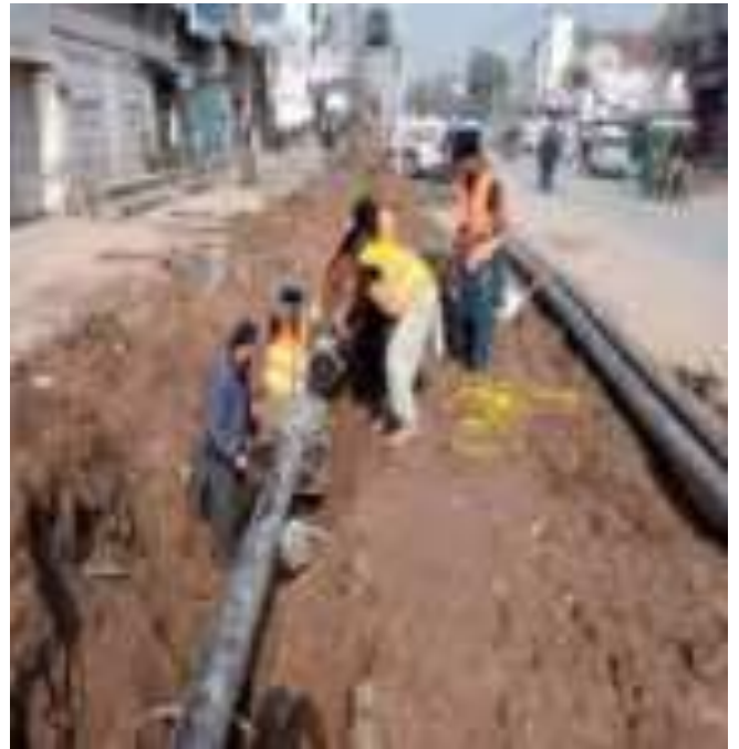
Laying of Water Supply Pipe
