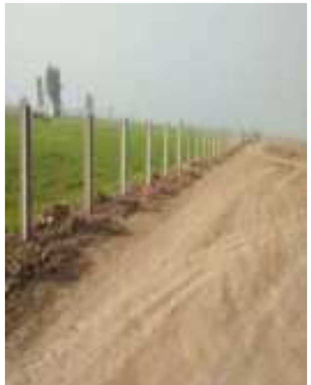
Boundary Wall Fence Post Installation in Progress
