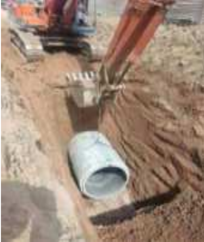
Laying of Sewer
