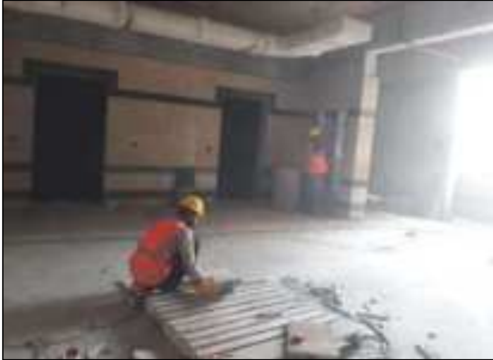
use of PPEs on site
