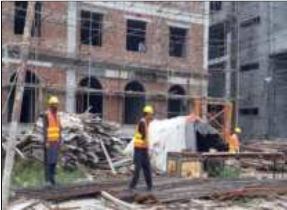
Figure: A use of PPEs on site 16-12-2022
