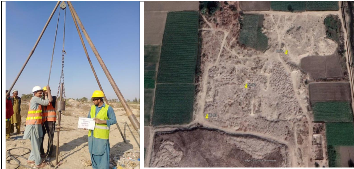
Figure 6-27 Borehole Drilling and locations at the MRF Site
