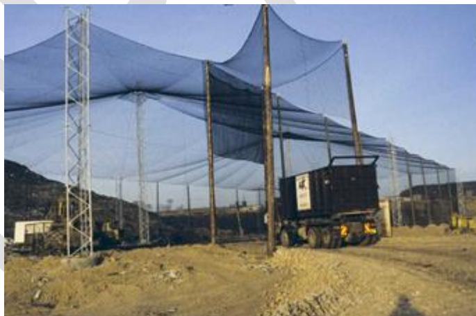
Example of a bird netting enclosure at an active tipping face on a landfill site
