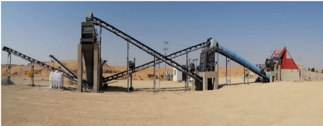
Figure 3-4: C&D recycling plant at proposed landfill site
